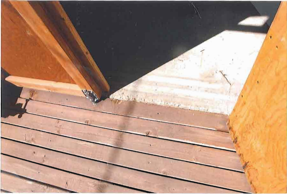
pre-existing concrete pad
