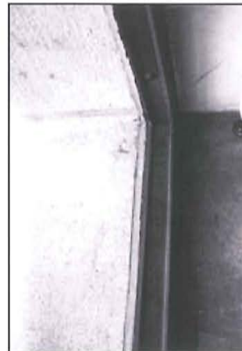
This is a successful replacement in kind of the deteriorated frame shown above. Photo: Henry Chambers, AIA.
