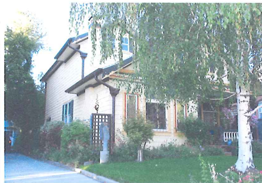
Front of house. 1221 4 th Ave.
