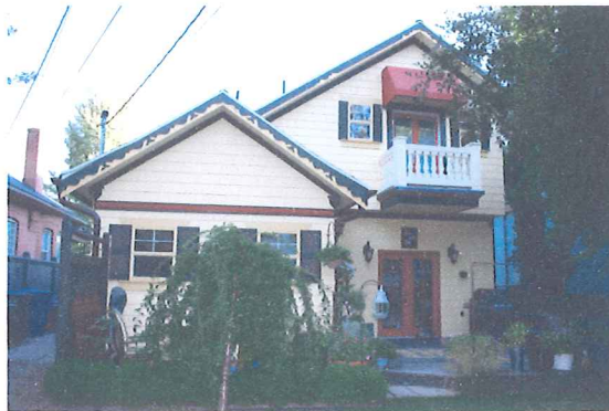
Back of house Showing 8/12 roof pitch.
