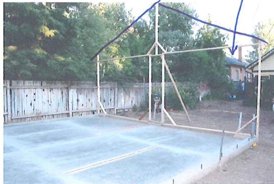
View South/East showing location of garage in proximity to east neighbor. *
