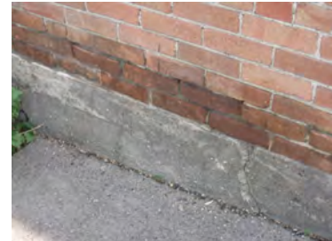
A concrete foundation at 422-426 N 300 West.
