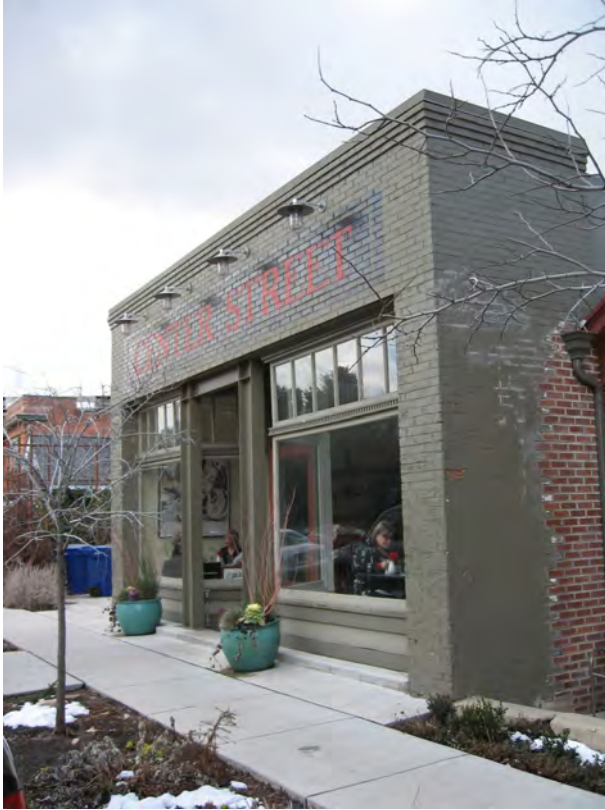
The building at 271 N Center Street has been preserved and rehabilitated as a restaurant.
