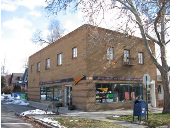
This building was designed with simple detailing ca. 1930 and has rectangular steel casement windows and original display windows (702 E. K Street).
