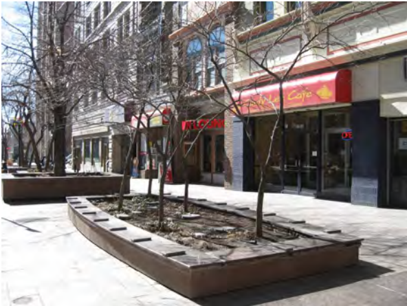
Added planter box and street trees in the 200 block of S Main Street.
