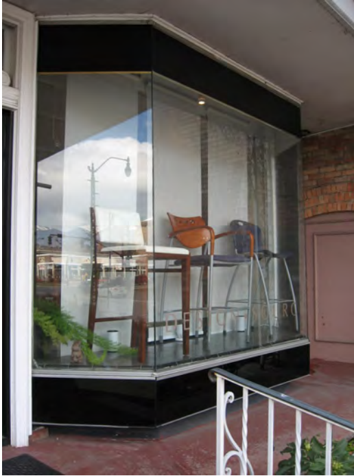
Few historic commercial buildings are located along South Temple but at 432-434 S Temple is a building with an intact ca. 1930s Carrara glass storefront.
