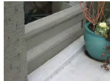
This rebuilt bulkhead at 361 N Center Street is a good example of in kind replacement.
