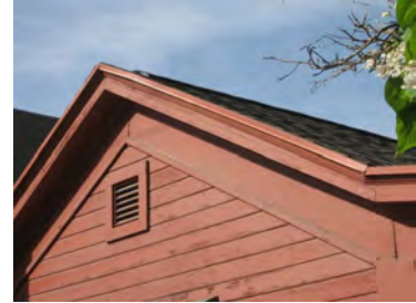
Maintain historic roof shapes (271 N Center Street).
