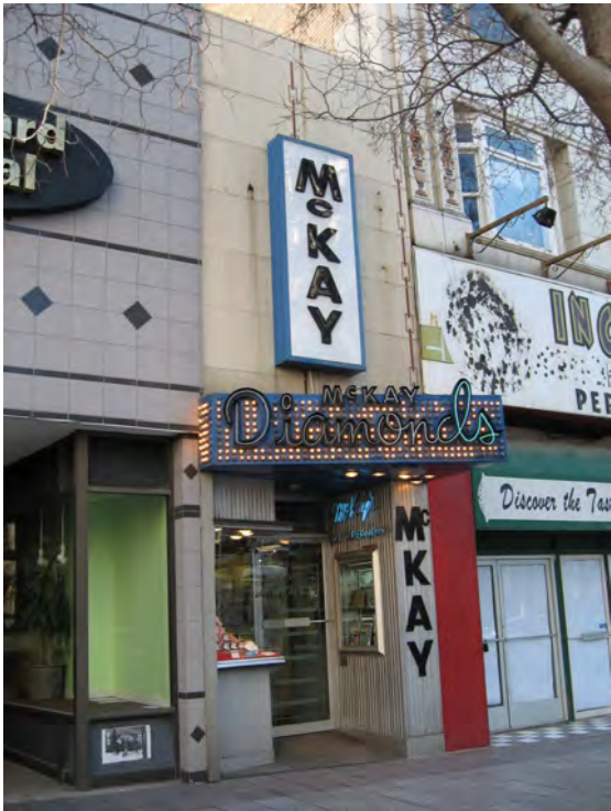
The McKay Jewelry Company at 157 S Main Street occupies a building completed ca. 1950 and features a restrained upper façade and original aluminum and glass storefront.
