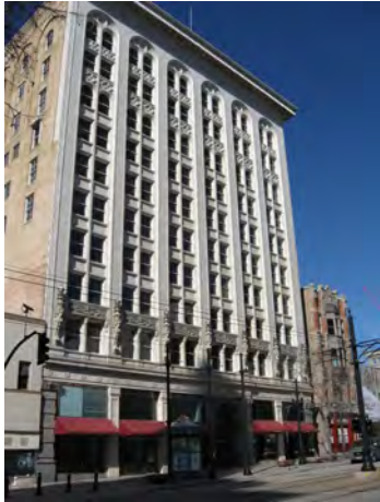
The Kearns Building at 136 S Main Street is representative of the Sullivan style.
