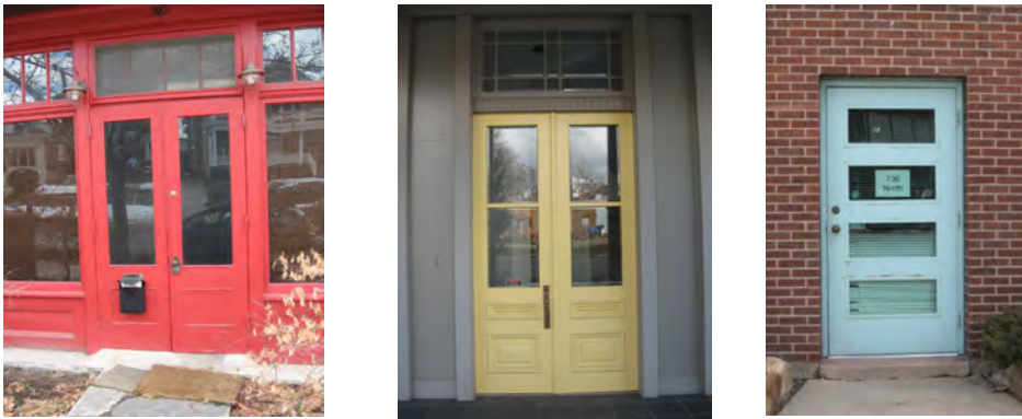
Salt Lake City's commercial buildings have a variety of doors and entrances: Original double doors at 361 N Main Street (left) and 740 2nd Avenue (center), and an original steel door at 736 N 300 West (right).
