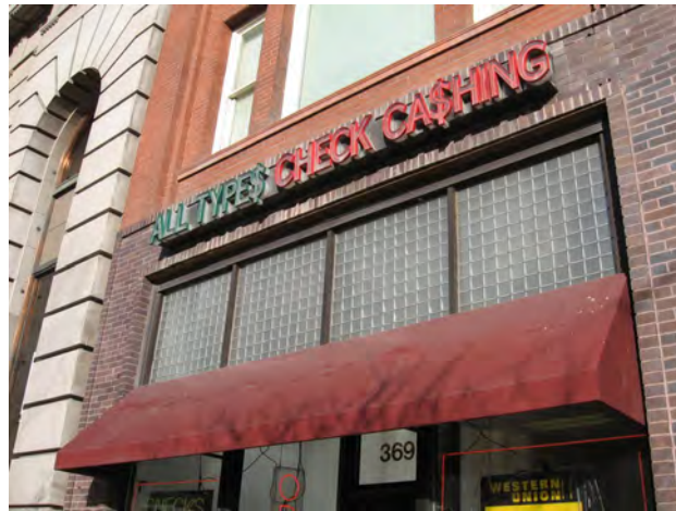
The distinctive Luxfer glass transom on the New Grand Hotel at 369 S Main Street should not be removed or concealed.
