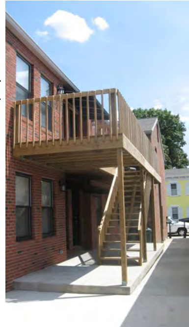
Rear decks of wood construction are appropriate on rear elevations not readily visible from the street.
