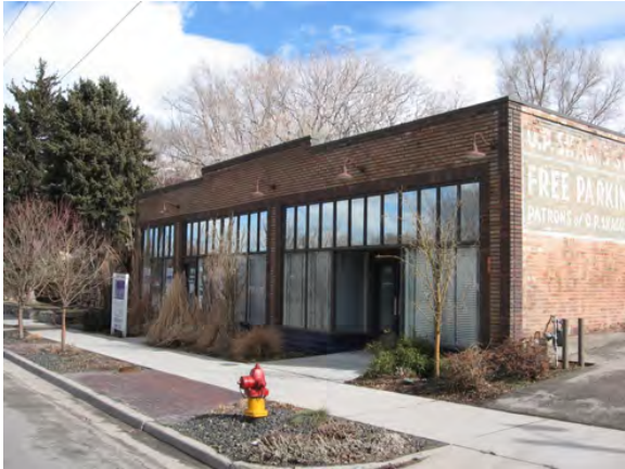
The building at 422-426 N. 300 West is a good example of a neighborhood shopping commercial building.
