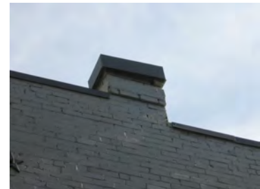
Original chimney, 68 N 'K' Street.
