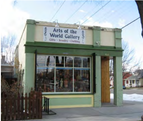
A good example of a One-Part commercial block is the building at 802 S 600 East.
