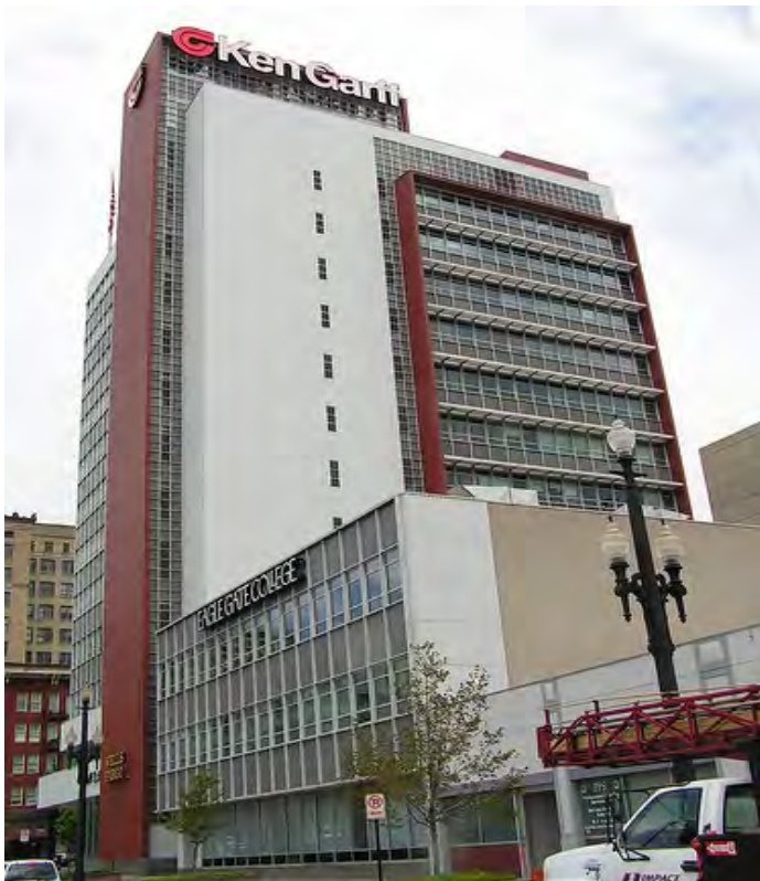
The First Security Bank Building at 405 S Main Street was built in 1955 and features an exterior curtain wall of glass, aluminum, and enameled porcelain panels.
