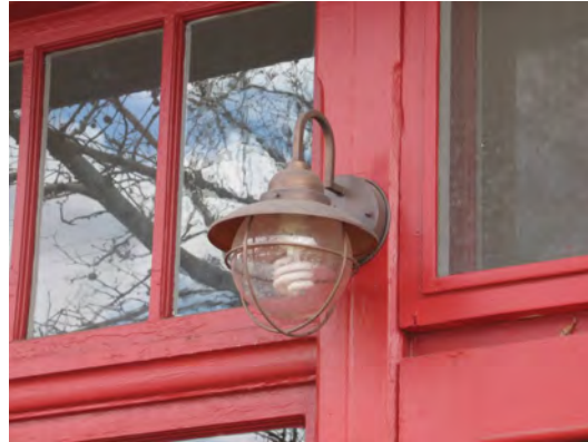
Good lighting choices for historic buildings should be simple and unobtrusive, such as the example shown above at 361 N Main Street.
