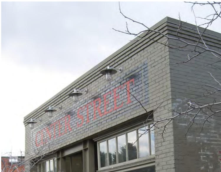
Signs above the storefront are historically correct locations for sign boards or painted wall signs such as at 271 N Center Street.
