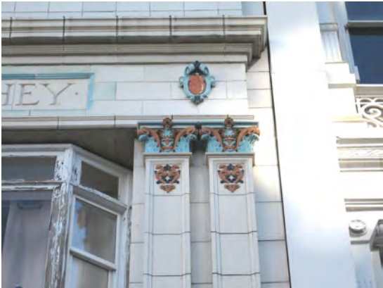
Downtown contains buildings with notable detailing such as the terra cotta façade at 159 S Main Street.
