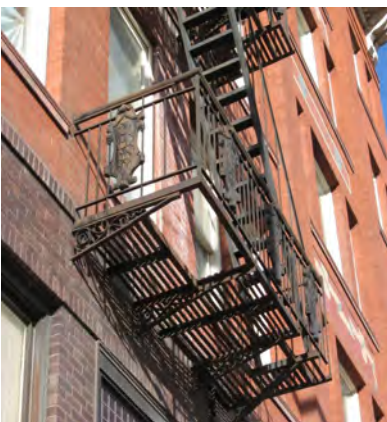
At left: Historic fire escape at 379 Main Street.
