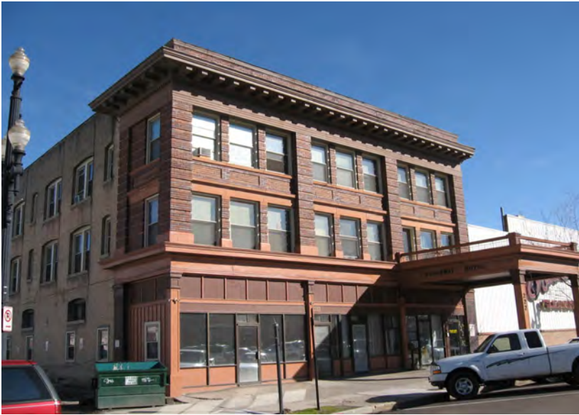
Pilasters divide the upper façade at 222 W 300 South and present a balanced and symmetrical appearance.
