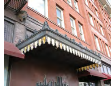
An example of a metal awning on the New Grand Hotel at 369- 379 S Main Street.
