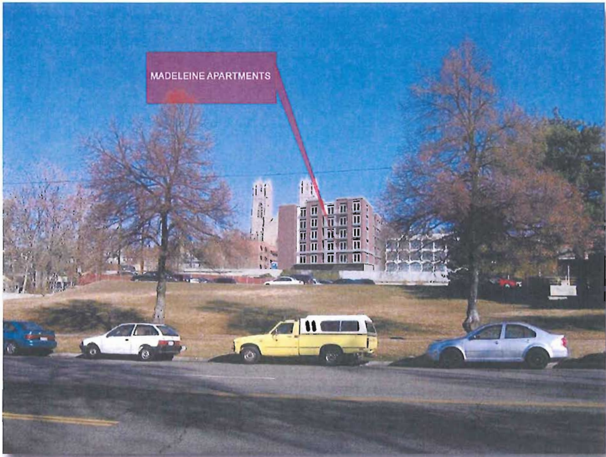
View along 400 South at the back of Madeleine Apartments.
