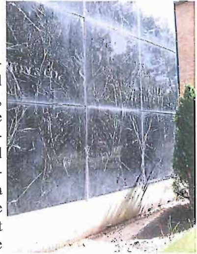
Marble paneled veneer on the main façade at 641-645 E South Temple Street, which was built in 1957.
