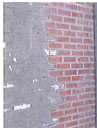
Leave historic brick unpainted (271 Center Street).
