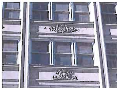
Rows of windows separated by decorative spandrels reflect the Sullivan style in the McIntyre Building at 68-72 S Main Street.
