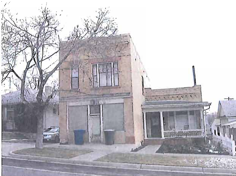
This house store at 228 N 'B' Street demonstrates the compatible, yet distinct commercial and residential units of this building form.
