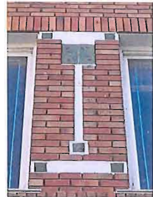
Preserve and maintain architectural details, 145 S State Street.
