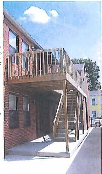
Rear decks of wood construction are appropriate on rear facades not readily visible from the street.
