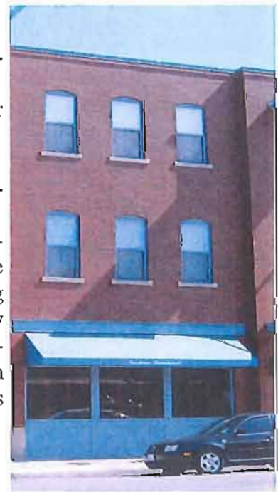
New construction such as illustrated above should have windows and storefronts in keeping with traditional designs and detailing.
