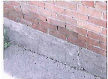
A concrete foundation at 422-426 N 300 West.
