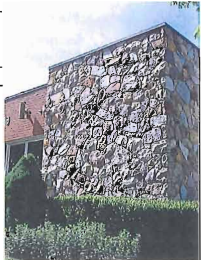
This stone veneer corner bay at 633 E South Temple Street was built in 1960.
