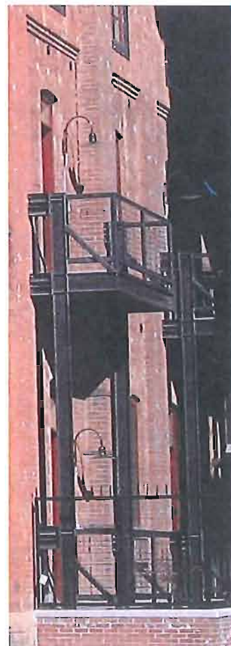
This metal fire escape has been appropriately added to the side elevation of the building.
