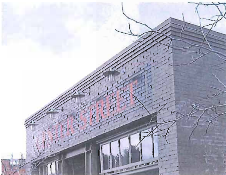
Signs above the storefront are historically correct locations for sign boards or painted wall signs such as at 271 N Center Street.
