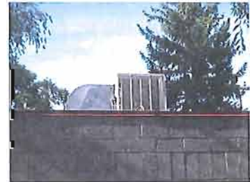
This roof mechanical system is set back so that it is not readily visible from the street.
