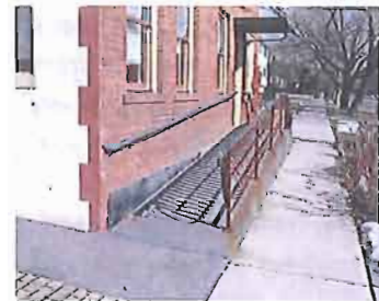
An appropriate access ramp at 569 E 2nd Avenue.
