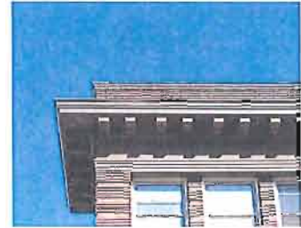
Historic cornices should be preserved and maintained (Broadway Hotel, 222 W 300 South).
