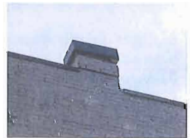
Original chimney, 68 N 'K' Street.
