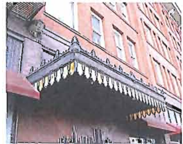
An example of a metal awning on the New Grand Hotel at 369- 379 S Main Street.
