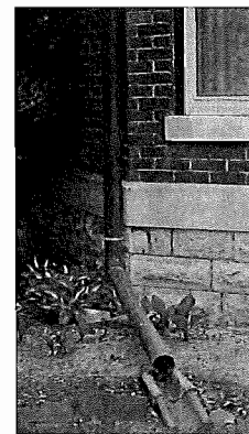
Appropriate downspout and splash block.
