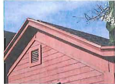
Maintain historic roof shapes (271 N Center Street).
