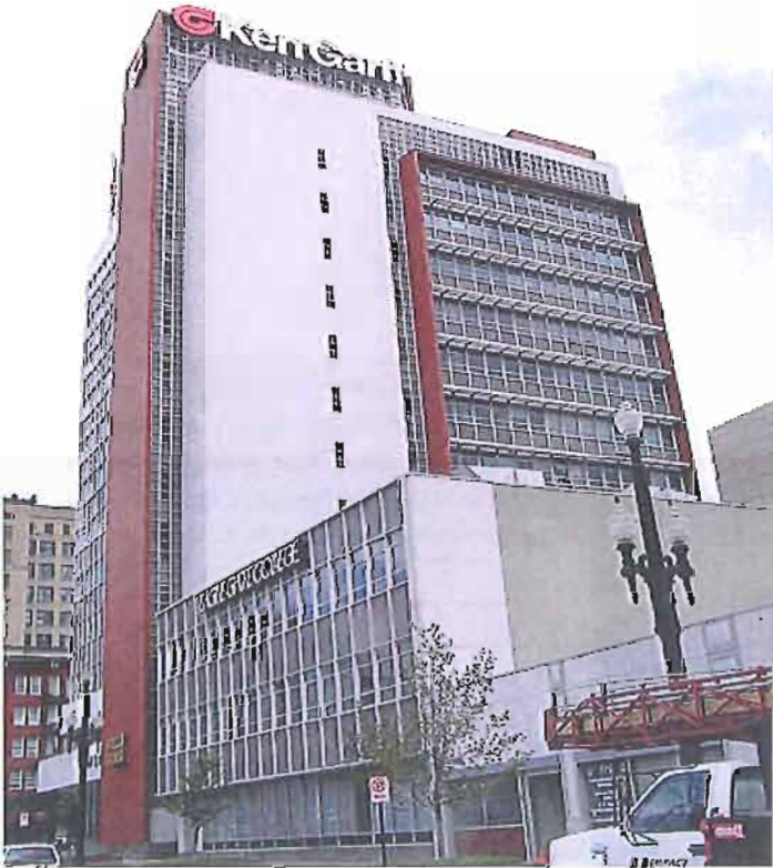
The First Security Bank Building at 405 S Main Street was built in 1955 and features an exterior curtain wall of glass, aluminum, and enameled porcelain panels.
