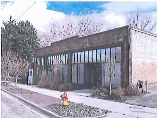
The building at 422-426 N 300 West is a one-story example of an enframed window wall plan with a simple brick surround around the storefront.
