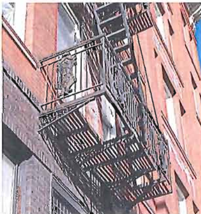
At left: Historic fire escape at 379 S Main Street.
