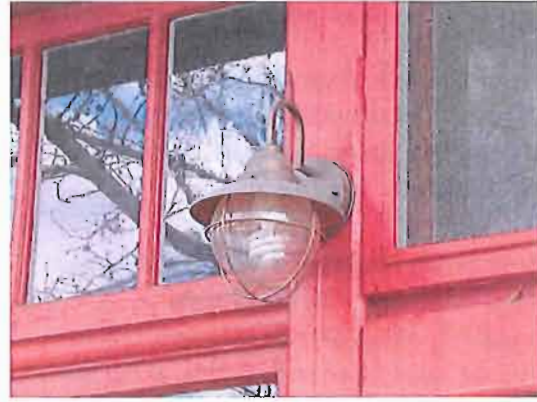
Good lighting choices for historic buildings should be simple and unobtrusive, such as the example shown above at 361 N Main Street.
