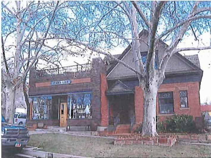
House stores can be found in a variety of styles and forms throughout Salt Lake City.
