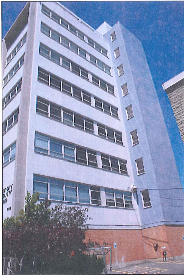
9 of 20. Pacific Northwest Pipeline Building; Camera facing north-northwest.
