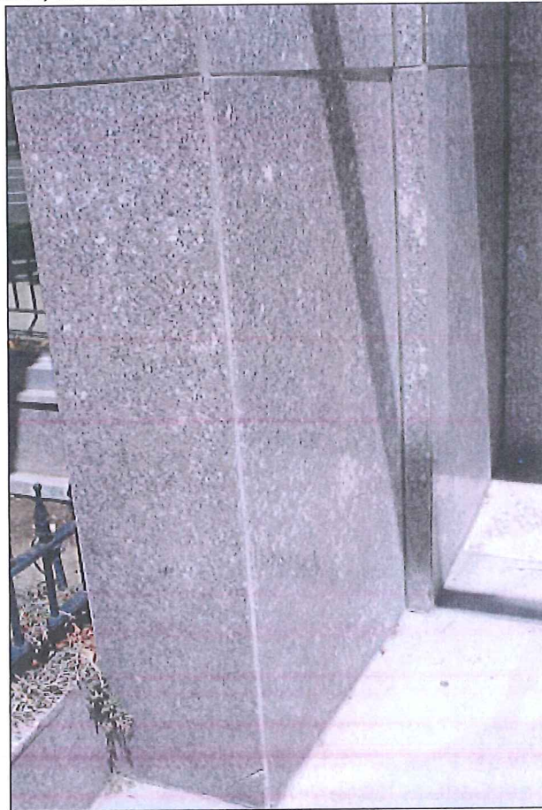
14 of 20. Pacific Northwest Pipeline Building; Thin stone veneer of enframed entry; Camera facing north.
