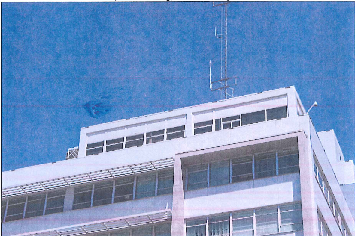
10 of 20. Pacific Northwest Pipeline Building; Penthouse office suite; Camera facing north-northwest.
