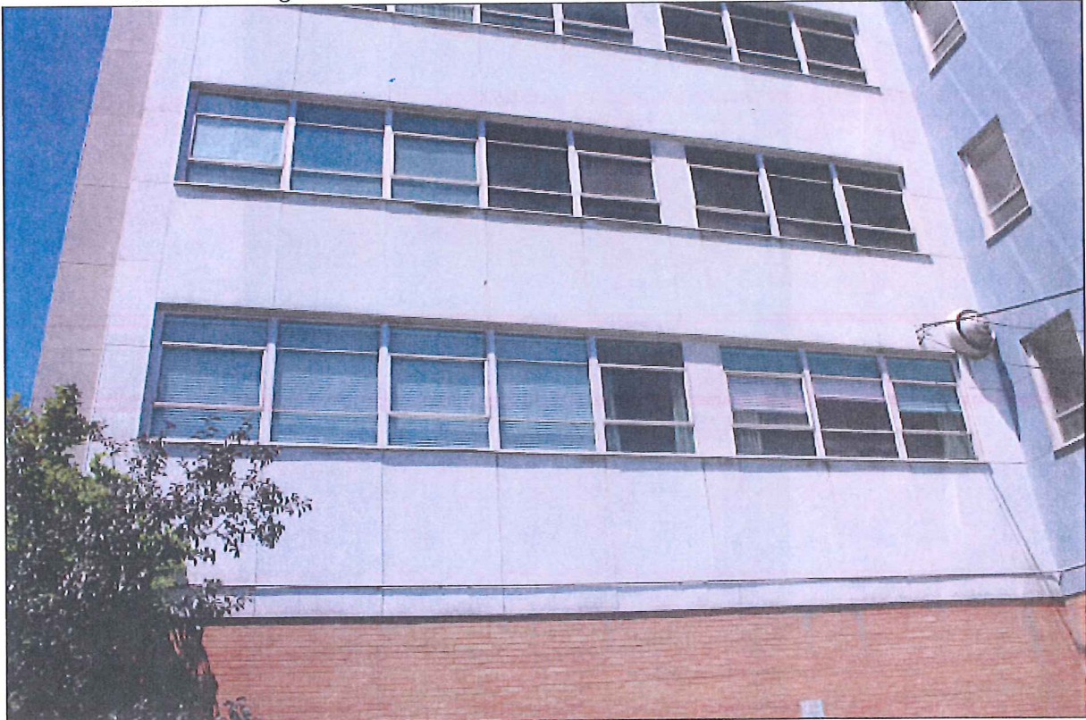
16 of 20. Pacific Northwest Pipeline Building; Example of window curtain wall construction on east elevation; Camera facing west.
