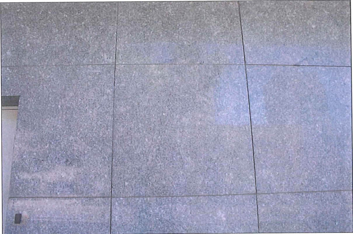
15 of 20. Pacific Northwest Pipeline Building; Close-up of thin stone veneer on west elevation; Camera facing east.
