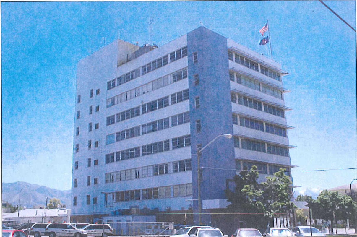
5 of 20. Pacific Northwest Pipeline Building; Camera facing southeast.
