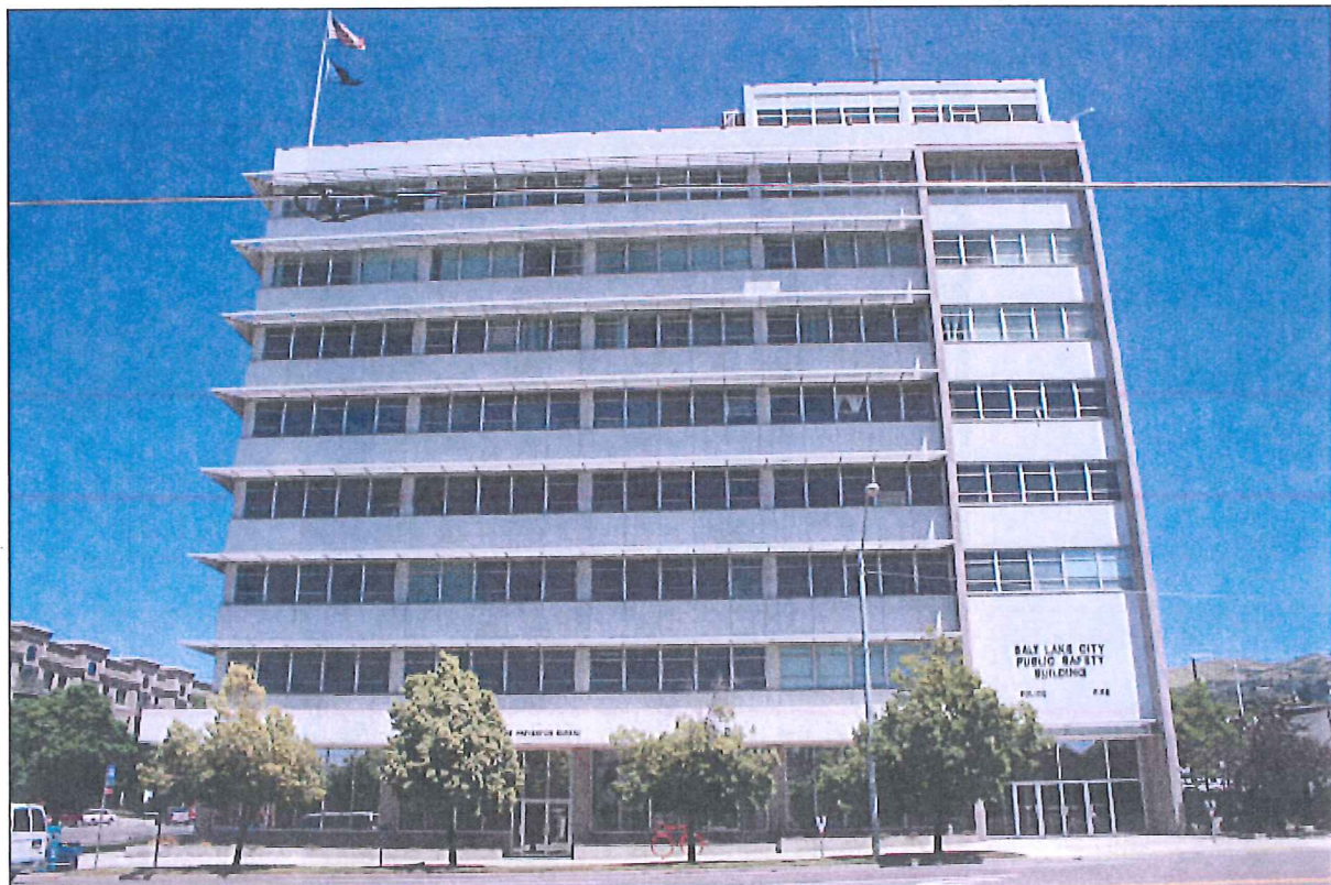
2 of 20. Pacific Northwest Pipeline Building; Camera facing north.
