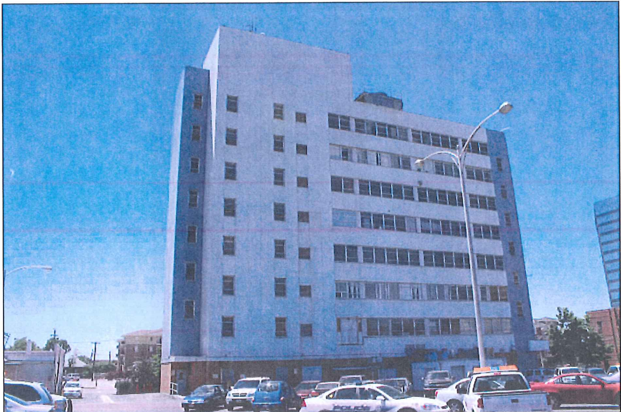
6 of 20. Pacific Northwest Pipeline Building; Camera facing south-southwest.
