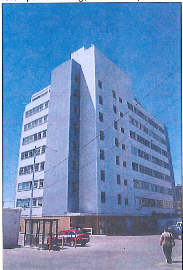
8 of 20. Pacific Northwest Pipeline Building; Camera facing southwest.
