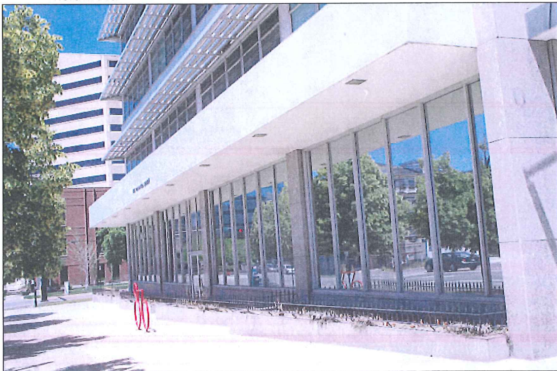
12 of 20. Pacific Northwest Pipeline Building; First (at-grade) story, south elevation window, projecting panel, and thin stone veneer detail; Camera facing northwest.
