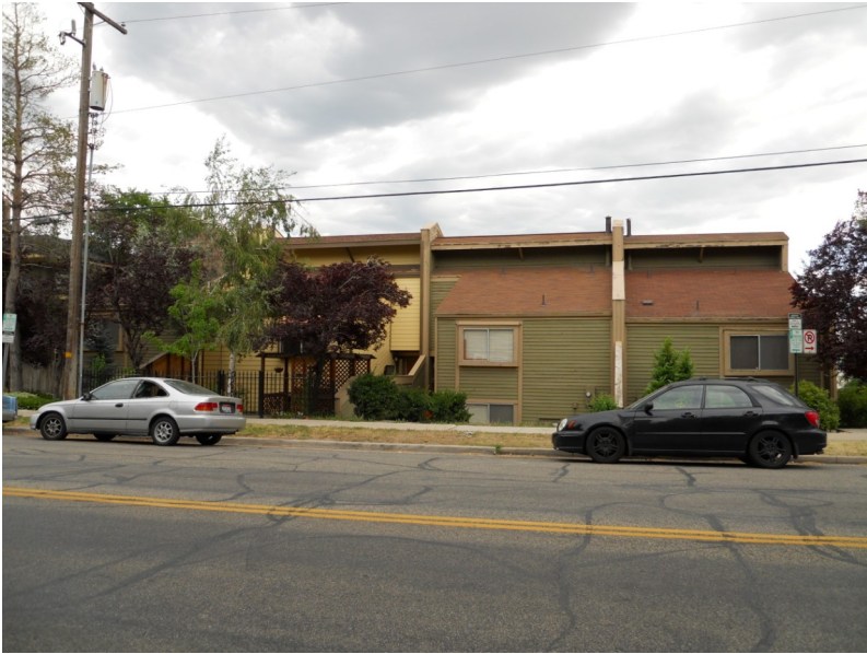
View of front façade from 1st Avenue
