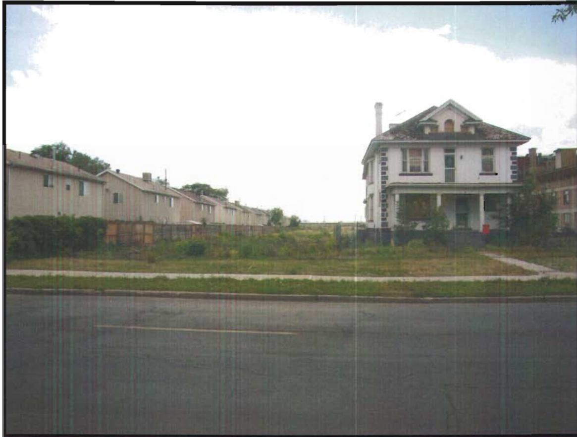
Westerly View of Adjacent Single-Family Development
