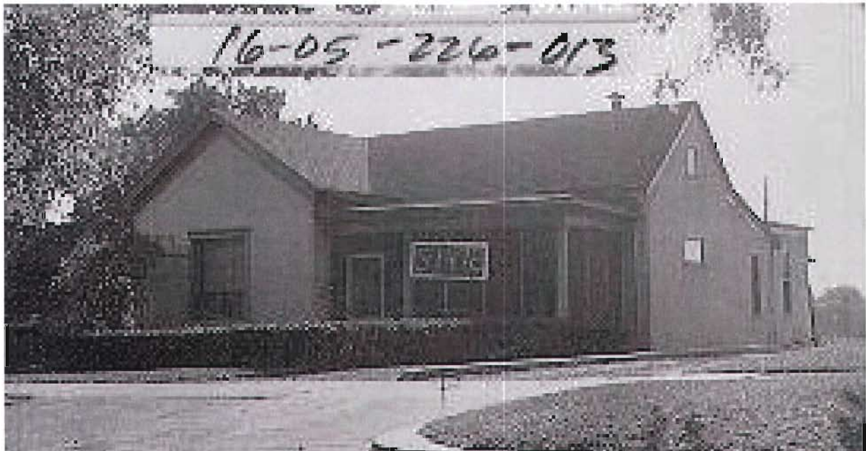
Historic Photo showing stucco siding. Date unknown.
