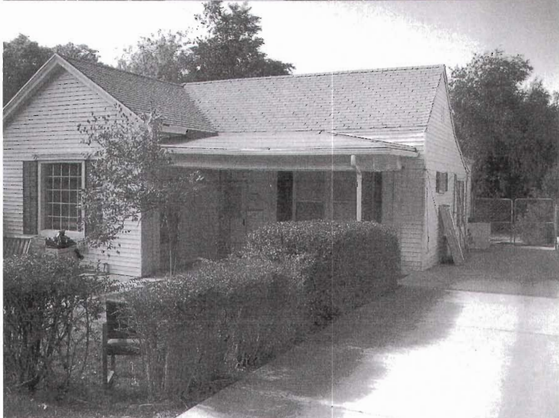
FRONT OF OWNER'S HOME. GARAGE WILL BE LOCATED AT THE BACK RIGHT SIDE OF LOT.
