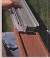
5. Slide bottom rail over the metal insert.
