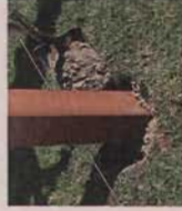
3. Set posts in concrete.
