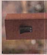
4. Install brackets using the TrexExpress™ installation tool.
