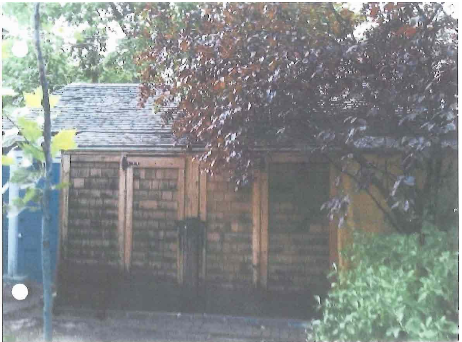
NORTH ELEVATION OF EXISTING GARAGE TO BE DEMOLISHED
