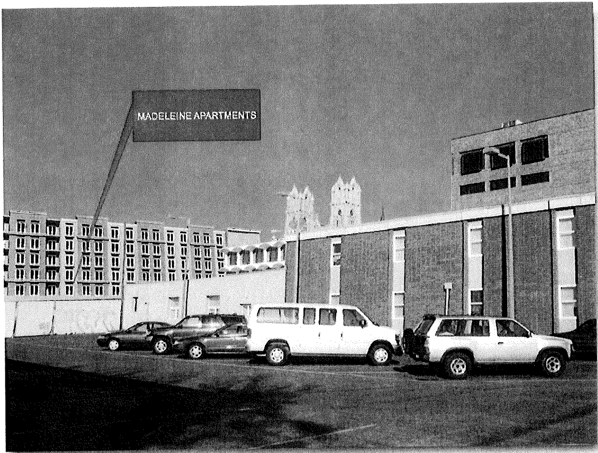
View from the parking lot at the back of Madeleine Apartments.
