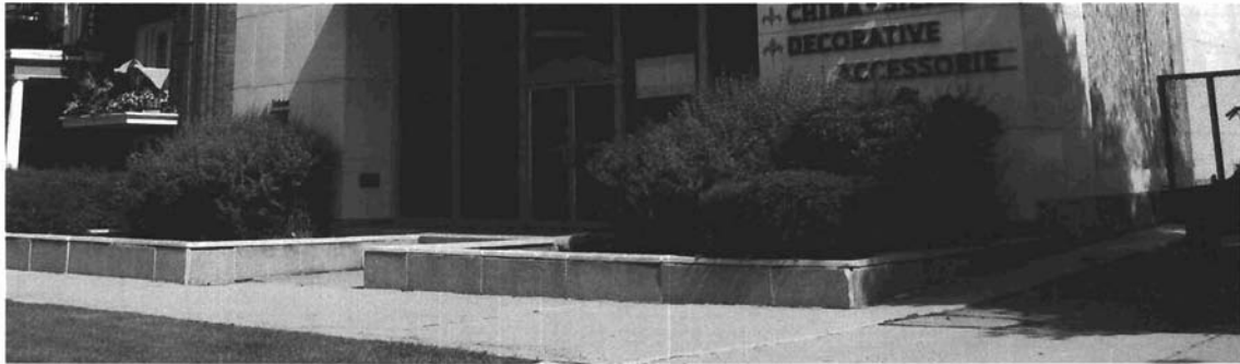
Masonry retaining walls in front of commercial buildings should be preserved and maintained such as this example at 445 E. South Temple Street.
