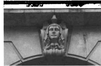
Details such as this decorative keystone at 32 Exchange Place should be preserved and maintained.
