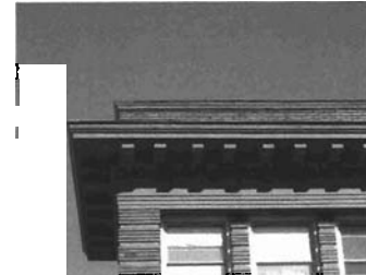
Historic cornices should be preserved and maintained (222 300 South).
