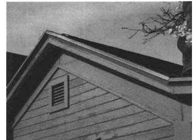
Maintain historic roof shapes (271 Center Street).
