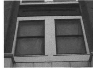
These one-over-one sash windows at 372 200 South are a good example of replacement windows. They match the historical design and configuration of the original windows.
