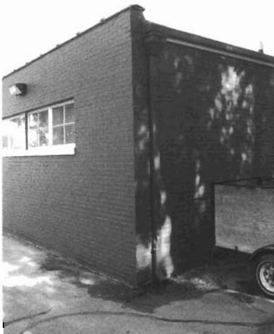
Appropriate rear gutter and downspout at 784 North 300 West Street .
