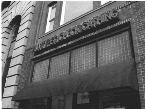
The distinctive Luxfer glass transom at 369 South Main Street should not be removed or concealed.
