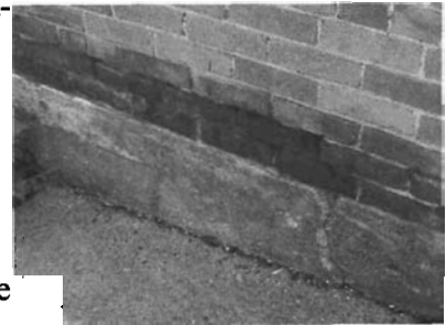
A concrete foundation at 422-426 North 300 West Street.
