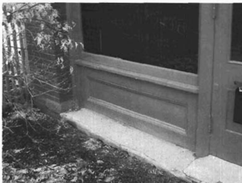
Original wood bulkheads such as those at 361 North Main Street (left) and 500 East Street (right) are significant parts of historic storefronts.
