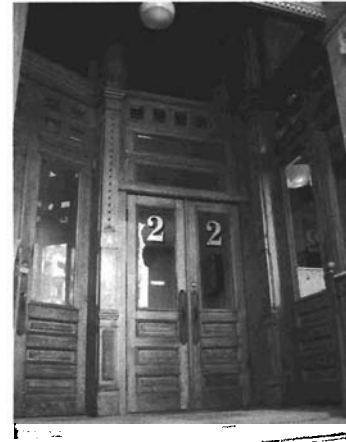
Original wood doors at 22 100 South.
