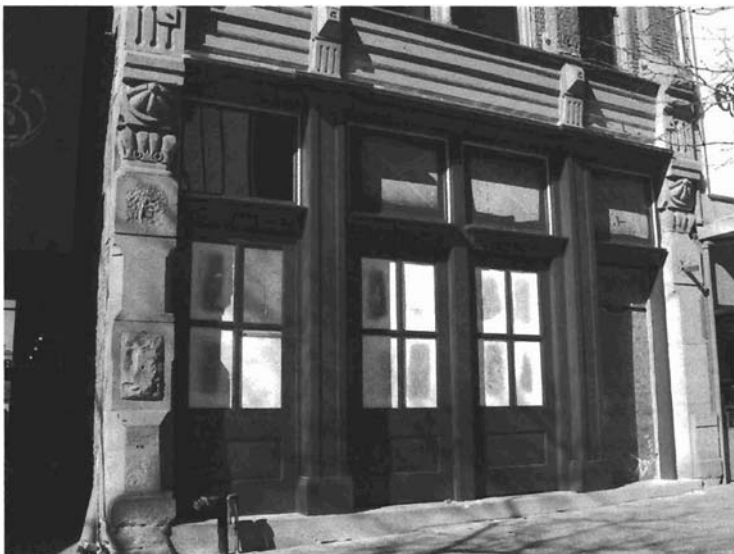
Maintain historic painted appearances (128 South Main Street).
