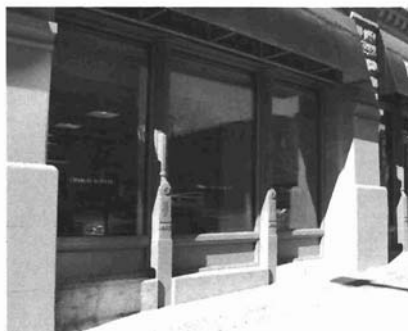
Cast Iron columns at 268 South State Street.
