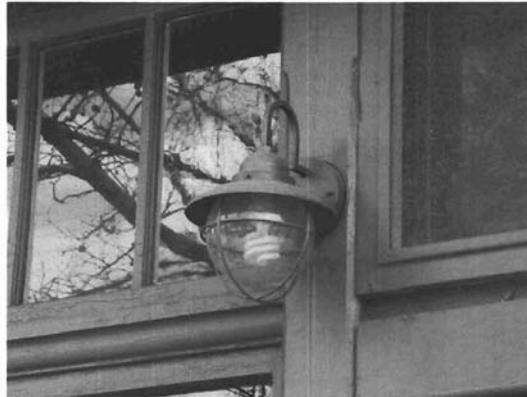
Good lighting choices for historic buildings should be simple and unobtrusive, such as the example shown above at 361 North Main Street.
