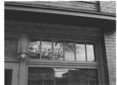
Original transoms enhance historic character and are important elements of commercial storefronts.
