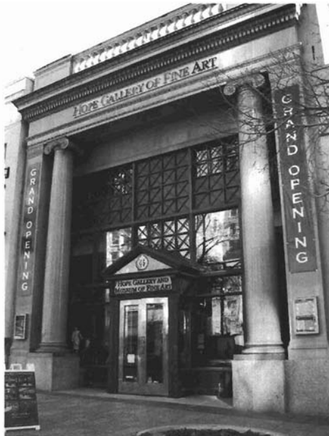
Classical columns and an accentuated entrance are key architectural features of the Gallery of Fine Art at 151 South Main Street.
