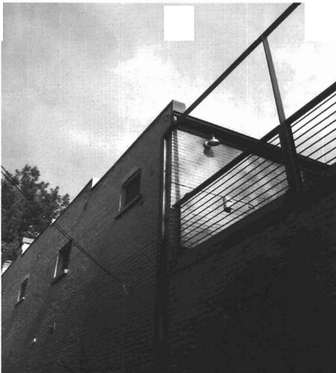
Decks such as this second floor addition at 68 North K Street are appropriate as long as they are not readily visible from the street and are located at rear facades.
