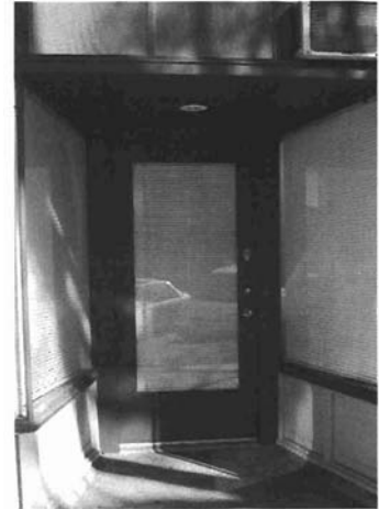
Rebuilt doors, such as this example at 428 300 South, should replicate the original as closely as possible.
