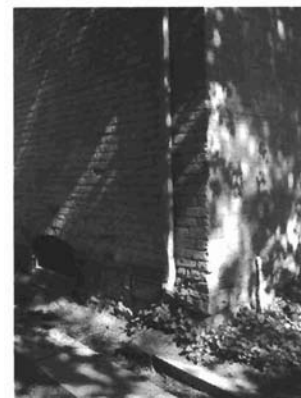
Appropriate downspout, Design and placement, 740 East 2nd Street.
