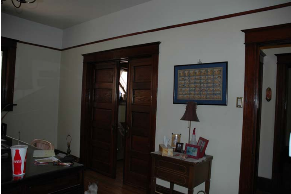
Photo No. 6: Interior detail
