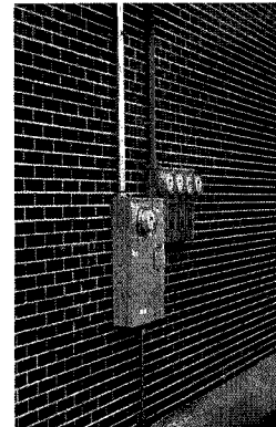
Meters at 39 North I Street are correctly placed on a non-primary elevation.
