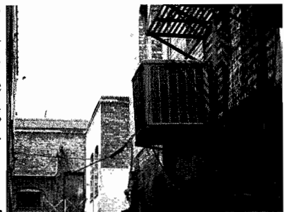
Heating and cooling units should be located at rear elevations such as shown here or on rooftop areas not visible from the street.
