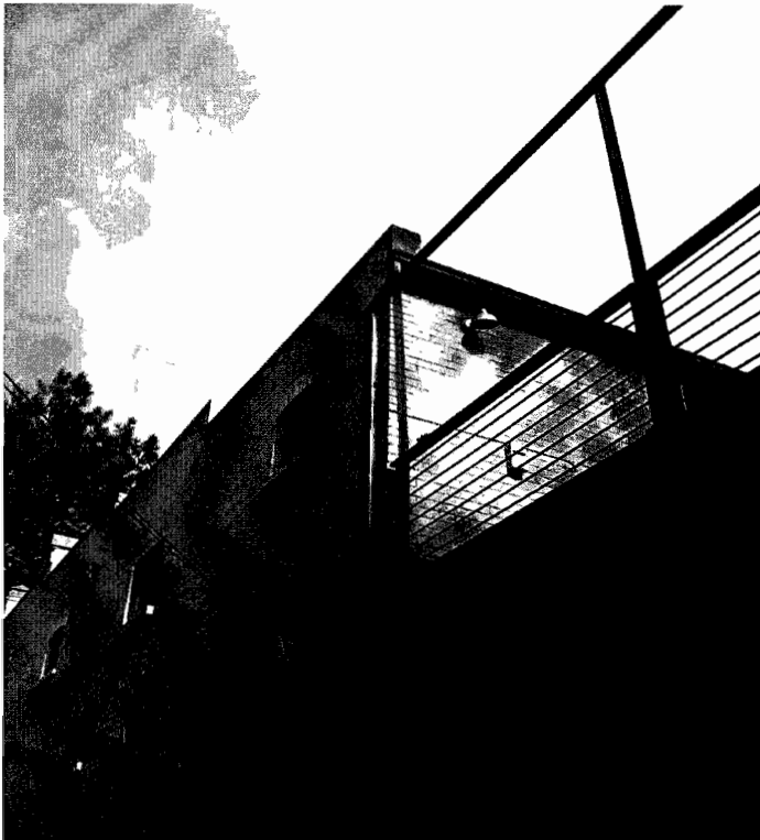
Decks such as this second floor addition at 68 North K Street are appropriate as long as they are not readily visible from the street and are located at rear facades.
