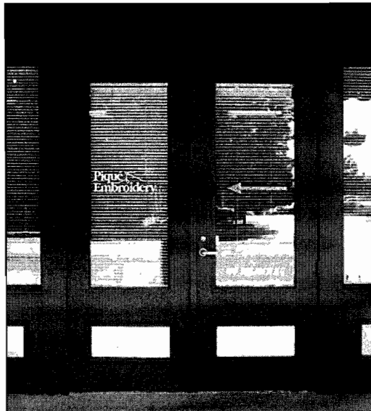
New storefronts should be designed with lever door handles and appropriate entrance widths.
