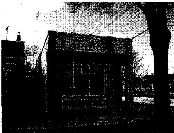
A good example of a One-Part commercial block is the building at 802 600 East.
