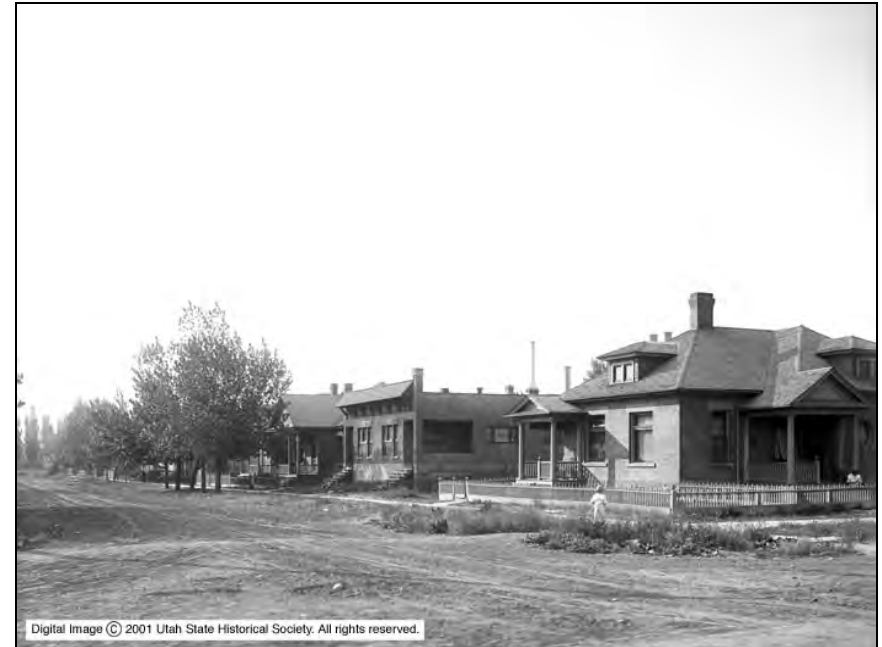
Figure 4. Euclid Avenue from 900 West as it appeared in 1914. Used with permission from the Utah State Historical Society, all rights reserved.
