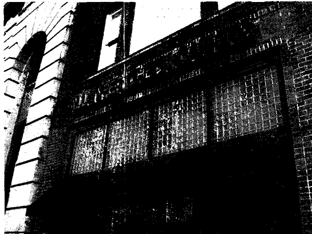
The distinctive Luxfer glass transom at 369 South Main Street should not be removed or concealed.
