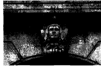
Details such as this decorative keystone at 32 Exchange Place should be preserved and maintained.
