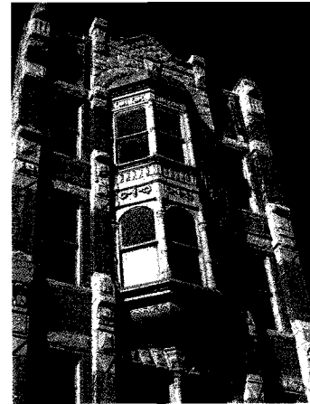
Historic masonry adds distinct character to buildings and should be preserved and maintained with proper care. (328 South Main Street)
