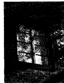
Casement window, 702 East K St.
