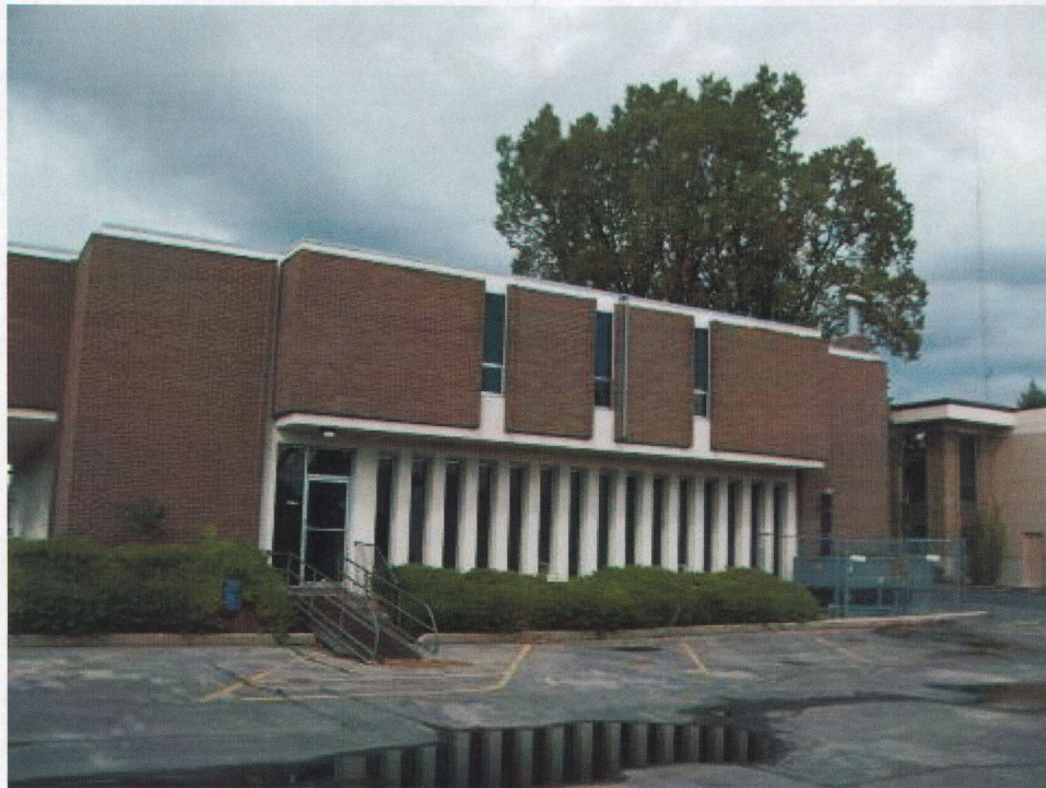
Rear entrance. The addition will extend outward from this rear wall over the parking spaces seen in this photograph.
