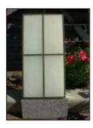
Walls: Remove existing exterior walls which serve as the back wall of the current exhibits and replace with CMU and Kalwall, a translucent wall material that will bring natural light into the interior exhibits and reduce the need for artificial light in the interior space. Replace existing doors into exhibits with insulated painted hollow metal doors and frames.
