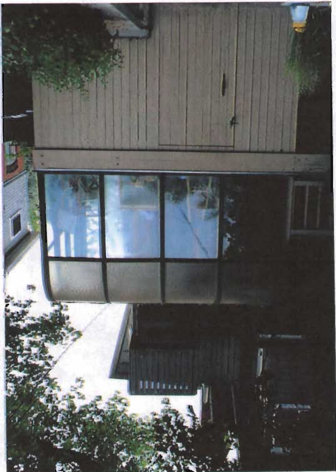
↓ Southeast corner to be removed - replaced
