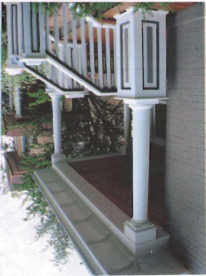
Detail to match - new remodeled porch
