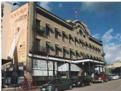
The New York Hotel at 60 West Market Street.
