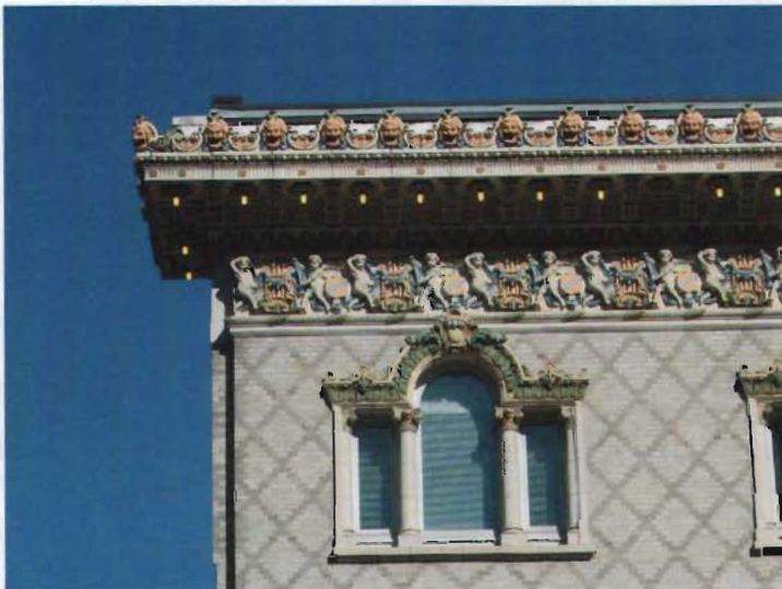
Architectural details of the Capitol Theater include an ornate cornice and decorative window hoods and surrounds.
