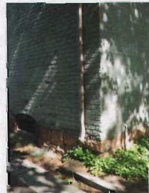
Appropriate downspout. Design and placement, 740 East 2nd Street.
