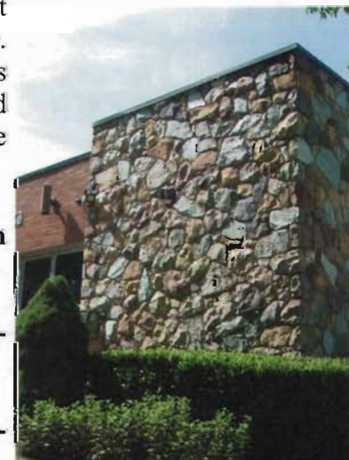
This stone veneer corner bay is at 633 E. South Temple and was built in 1960.
