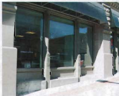
Cast Iron columns at 268 South State Street.
