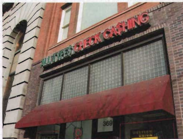
The distinctive Luxfer glass transom at 369 South Main Street should not be removed or concealed.
