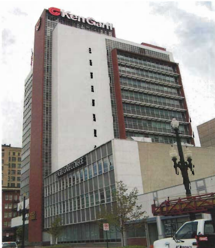
The First Security Bank Building at 405 South Main Street was built in 1955 and features an exterior curtain wall of glass, aluminum, and enameled porcelain panels.
