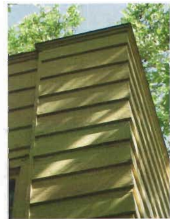
Original wood siding should be preserved and maintained. (801 East 1st Avenue).
