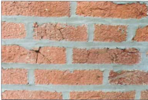
Hard mortars do not allow brick to expand and contract....
