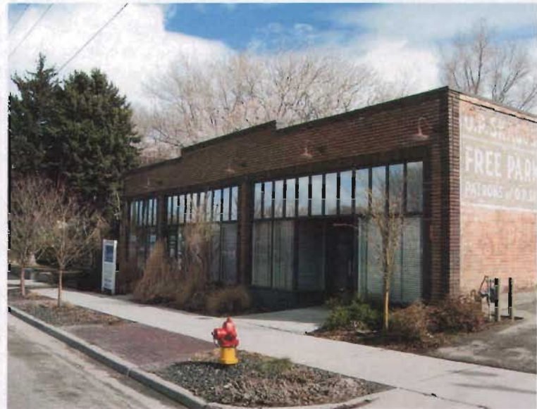
The building at 422-426 N. 300 West has been well preserved and retains much of its original storefront.
