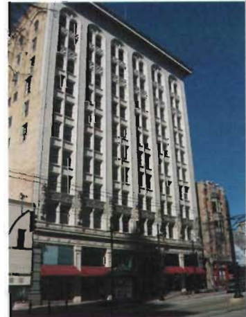
The Kearns Building at 136 South Main Street is representative of the Sullivan style.
