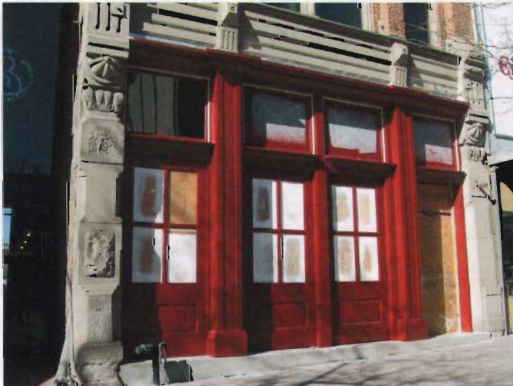
Maintain historic painted appearances (128 South Main Street).
