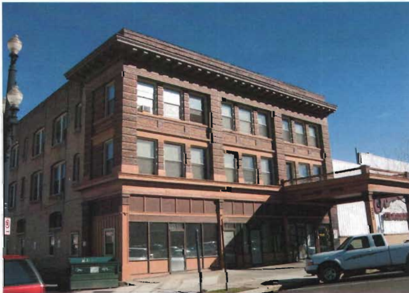
Pilasters divide the upper façade at 222 West Third South Street and present a balanced and symmetrical appearance.
