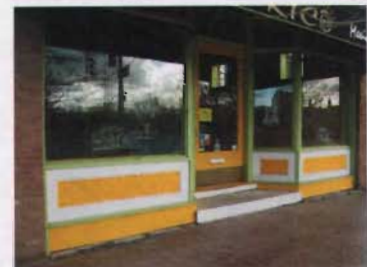
Original storefronts, such as those at 802 600 East (top) and 500 East Street (bottom), should be preserved and maintained.
