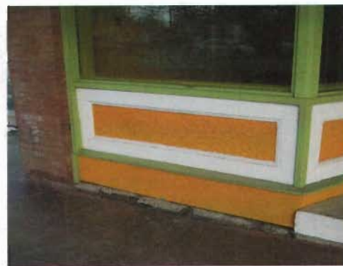
Original wood bulkheads such as those at 361 North Main Street (left) and 500 East Street (right) are significant parts of historic storefronts.
