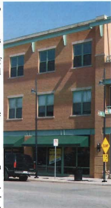
New construction should be designed with appropriately sized windows, storefronts and awnings as shown above.
