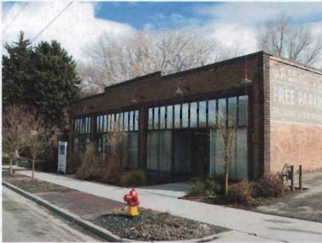
The building at 422-426 North 300 West Street is a one-story example of an enframed window wall plan with a simple brick surround around the storefront..
