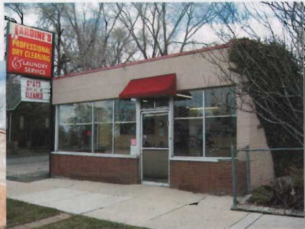
Neighborhood shopping center commercial buildings continued to be constructed into the 1940s in many residential areas of the city (442 North 300 West).
