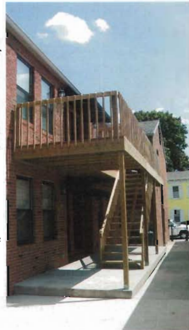
Rear decks of wood construction are appropriate at rear facades not readily visible from the street. .
