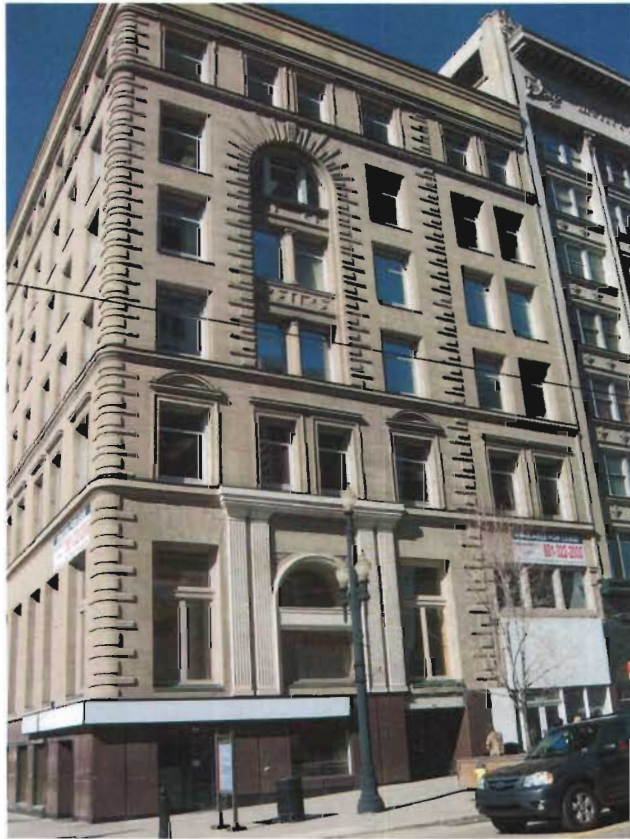
The McCornick Building at 74-78 South Main Street built in 1893 is an example of a three-part commercial building.. Although the first floor has been altered, it still retains its distinct treatment of designs on the first floor and rectangular windows on the seventh floor..
