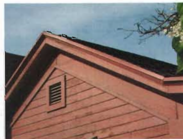
Maintain historic roof shapes (271 Center Street).
