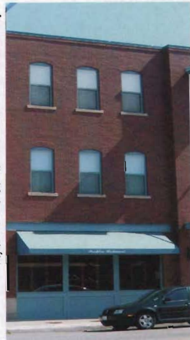
New construction such as illustrated above should have windows and storefronts in keeping with traditional designs and detailing.
