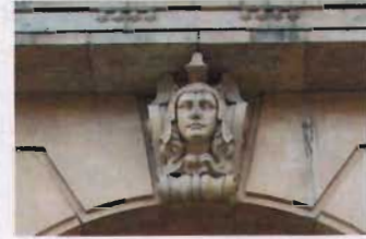
Details such as this decorative keystone at 32 Exchange Place should be preserved and maintained.
