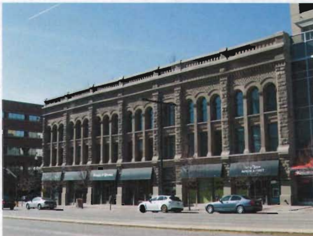
Rounded arches and textured masonry are common features of the Richardsonian Romanesque style.
