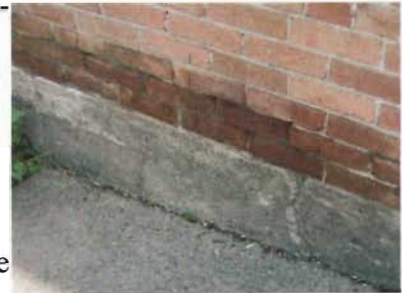
A concrete foundation at 422-426 North 300 West Street.
