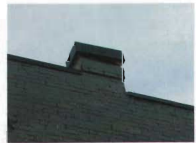
Original chimney, 68 North K Street.
