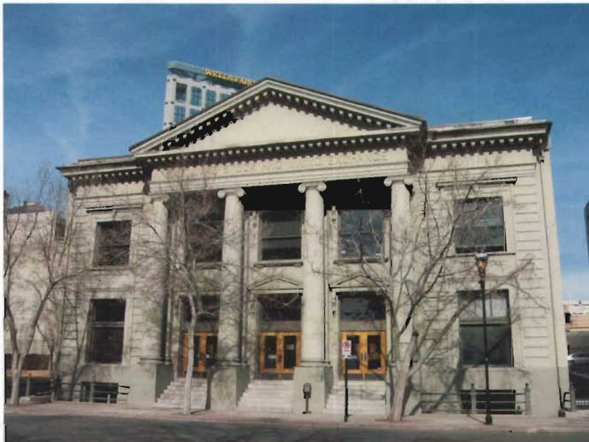
The Salt Lake Stock and Mining Exchange at 39 Exchange Place was built in 1908 and it retains much of its original design. The building's form is central block with wings while its architectural style is Neo-classical. The projecting central bay displays Ionic columns and a large pediment with modillion blocks.
