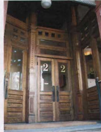
Original wood doors at 22 100 South.
