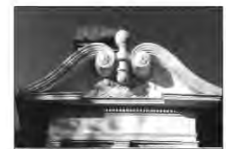
Replaces such as window hoods, brackets and columns are often painted with particular style and therefore their preservation is important.
