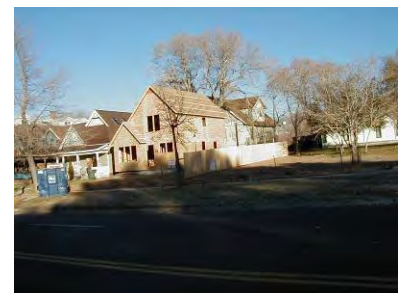
New house under construction.
