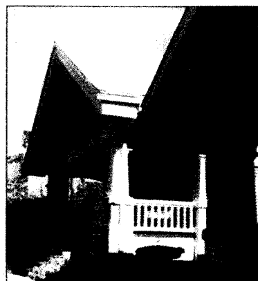
Supports for bungalow porches often have a sloped or "battered" design, which is a key feature.
