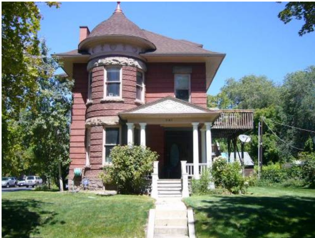
545 E 900 South (across Park Street)
