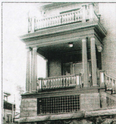
This classical detail porch includes paired Doric columns.
