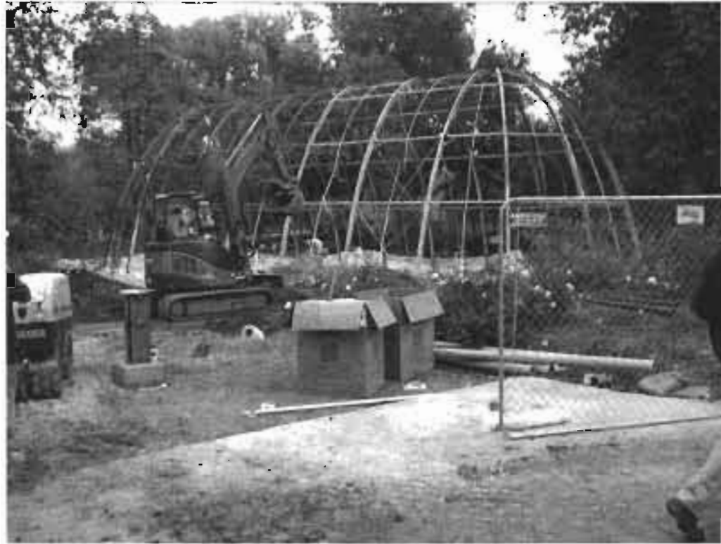
Existing Flight Cage during rehab
