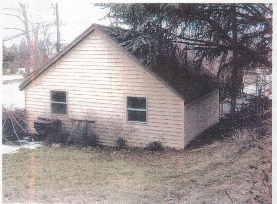
Back / West Side (from East)
