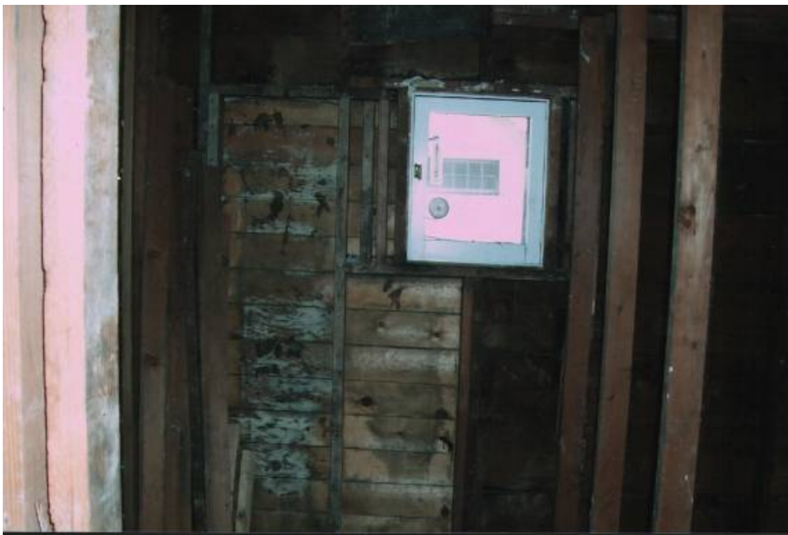
The lighter boards to the left are evidence of a hay loft door on the second floor, north side.
