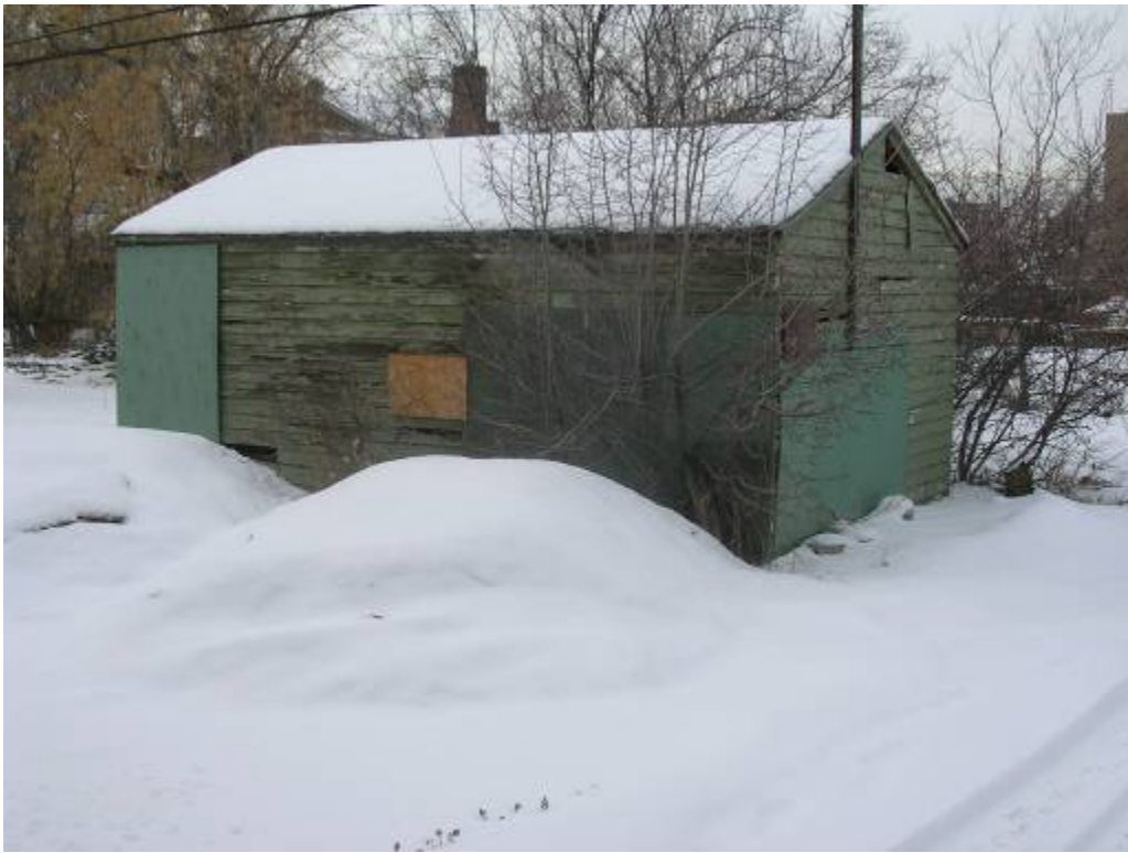
Accessory structure behind 46 South 700 East.
