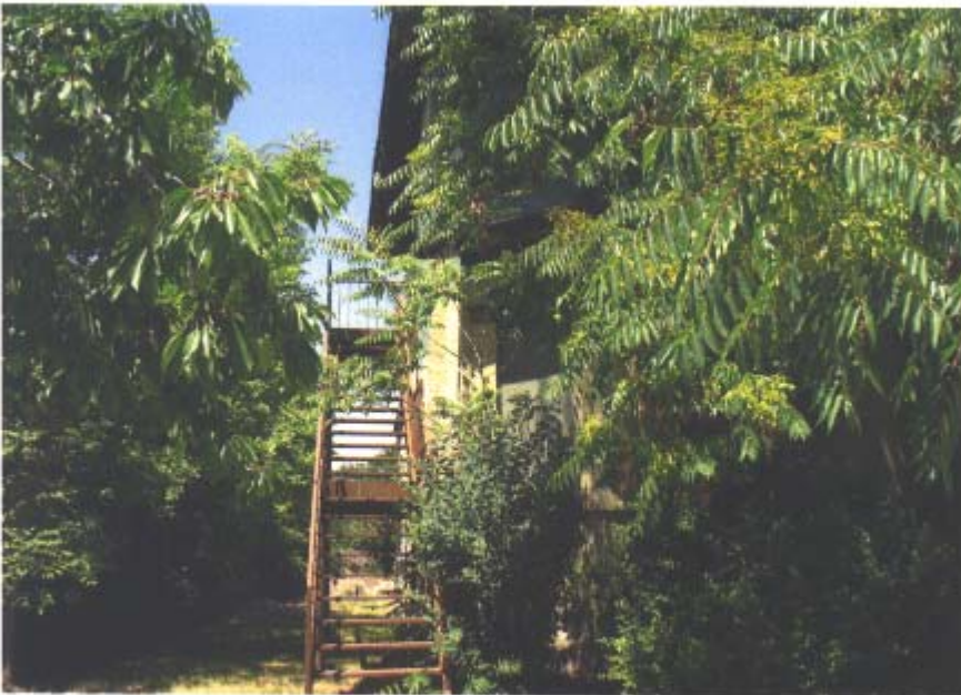
South side of property.
