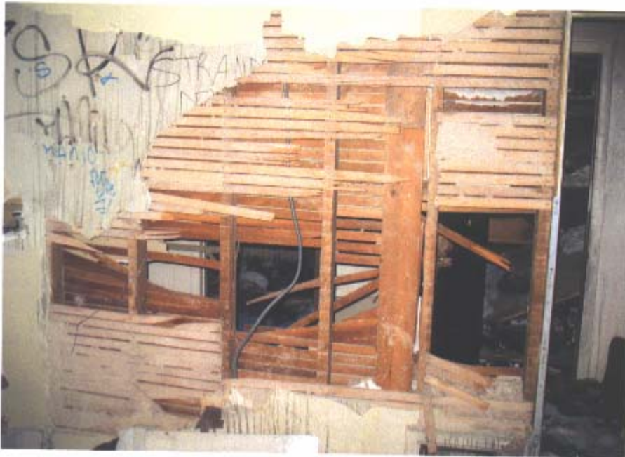
Opposite view of upstairs hallway wall.
