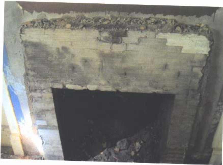
Close up of living room fire place.
