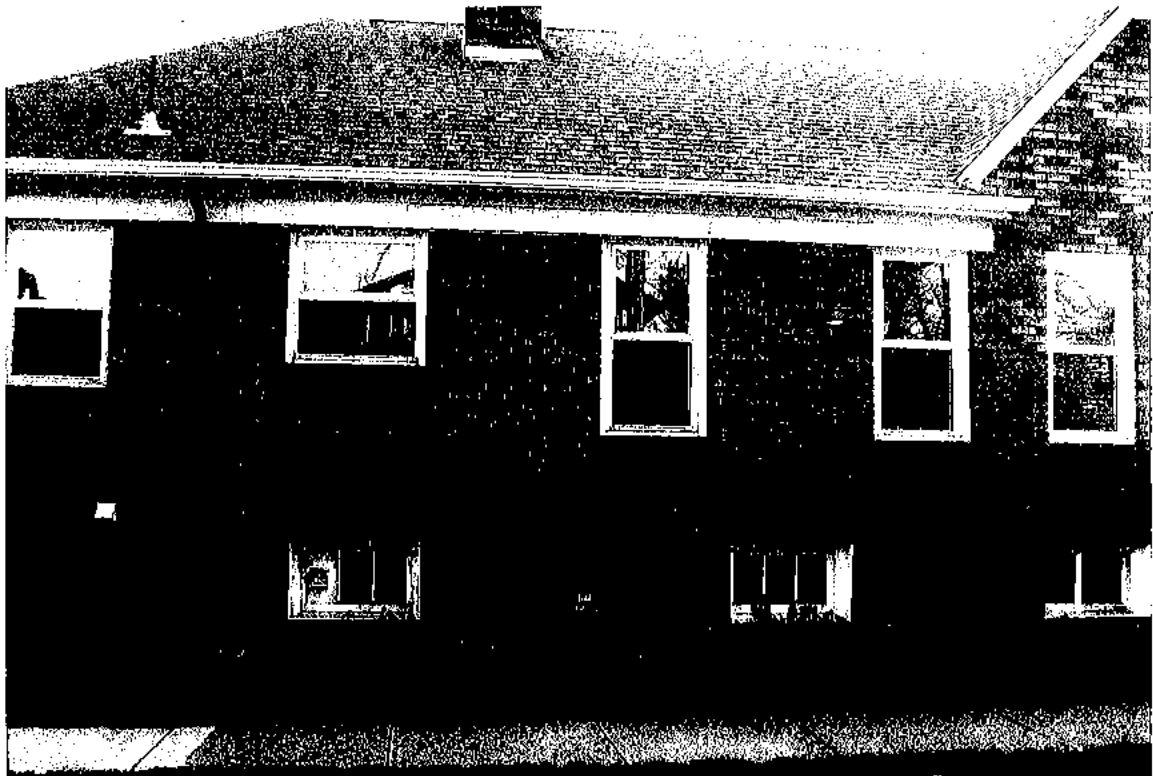
Vinyl window replacements on 3rd Ave Side
