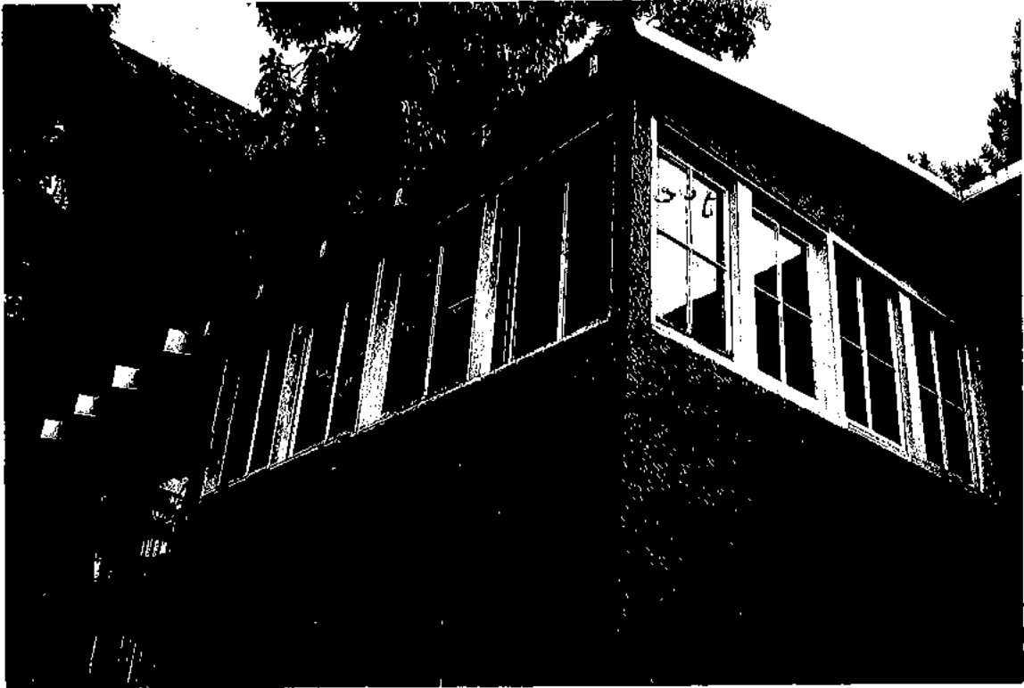
Sun room west side of building
