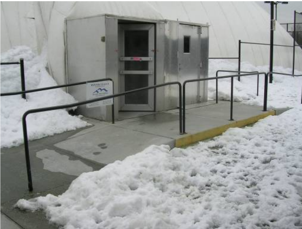
Seasonal entrance located immediately behind the tennis center building.
