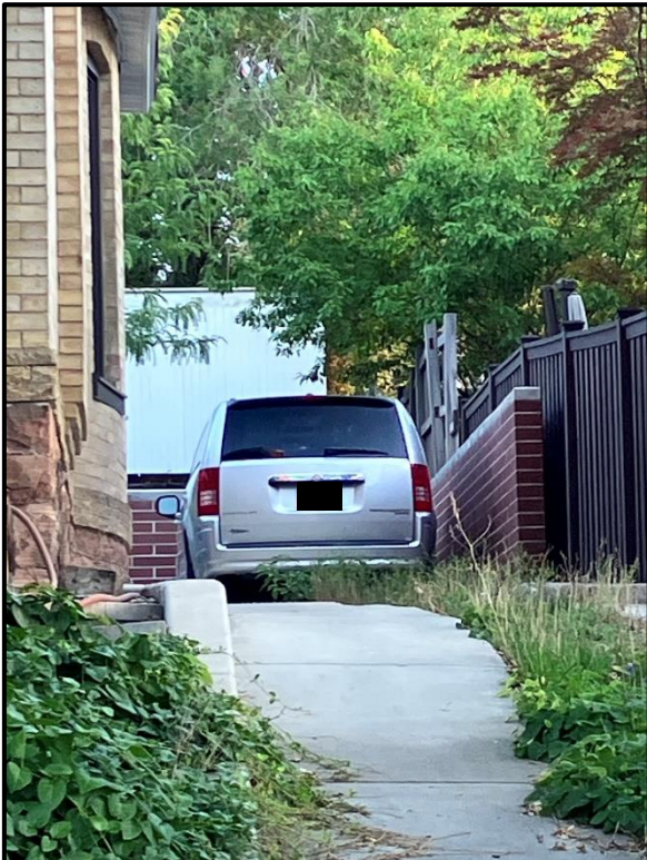
Brick retaining wall completed in 2016. This wall would need to be demolished to relocate the proposed accessory structure.
