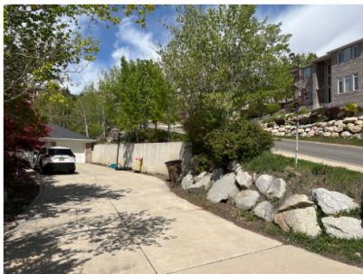
7' drop from front street to driveway (debris and hazard for individuals)
