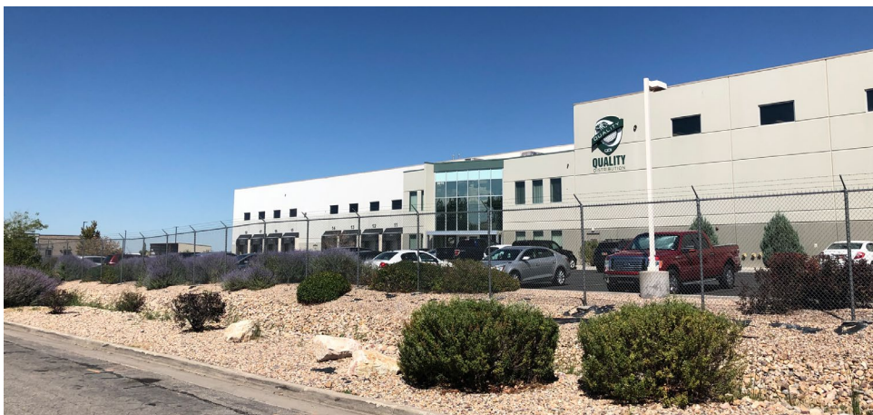
The property at 421 John Glen Rd. installed a 6’ fence – with barbed wire on top- prior to July of 2014.
