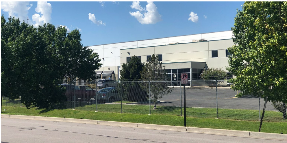
The property directly to the north -6010 W. Amelia Earhart Dr. – has a 6’ fence with barbed wire on top.
