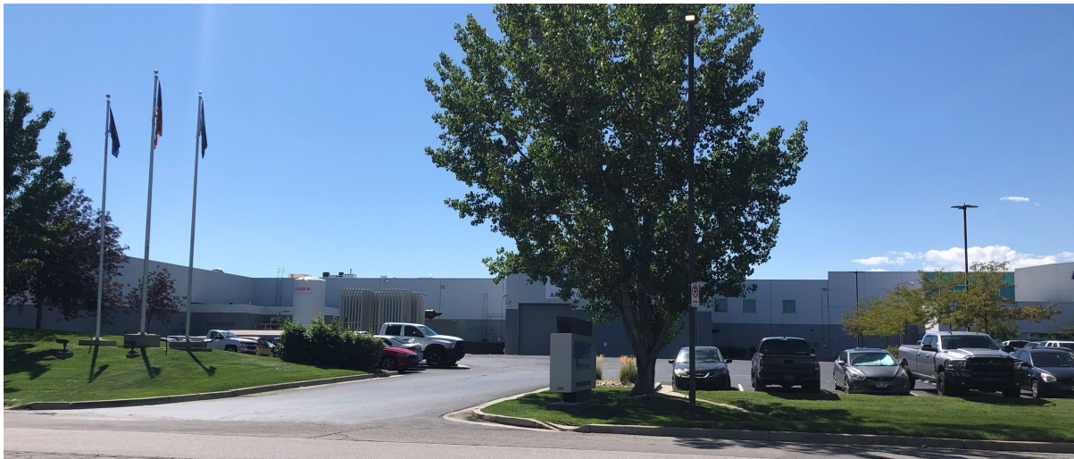
Northeast side of subject property.
