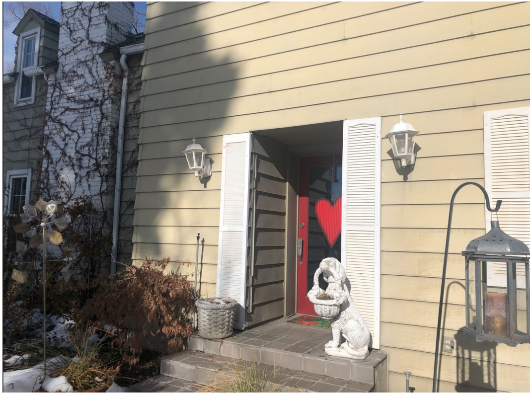
Existing front porch
