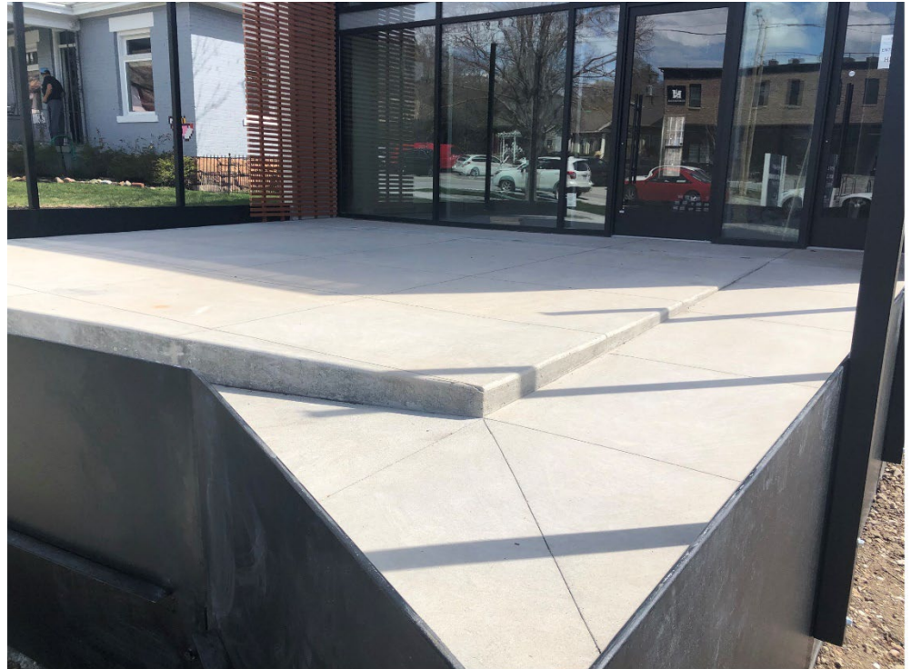
View of the front patio pad of subject building
