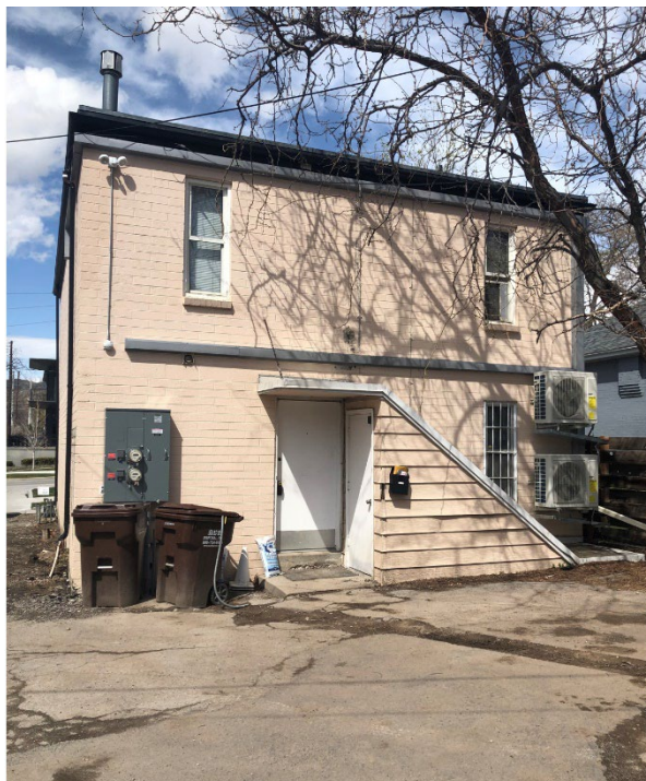
View of the subject building from the rear yard (looking north)
