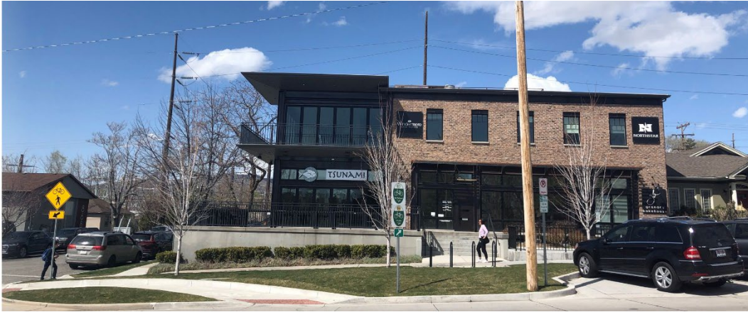
Building across the street to the north (restaurant use)
