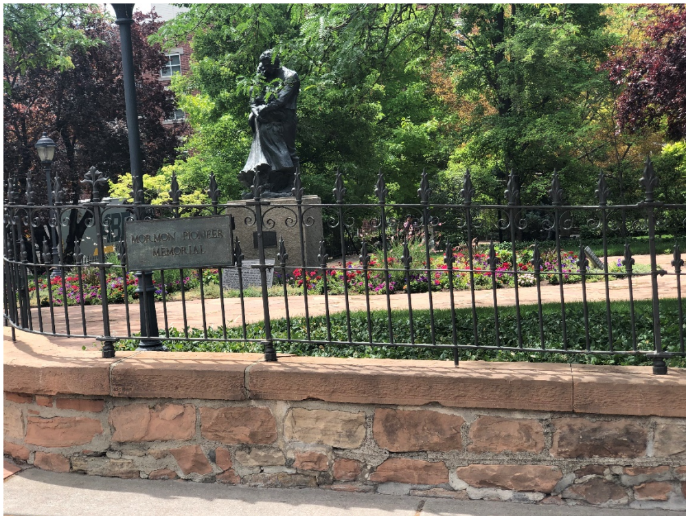
Existing fence along 1 st Avenue. The retaining wall and proposed fence will have a height of approximately 7 FT at the front property line along 1 st Avenue.
