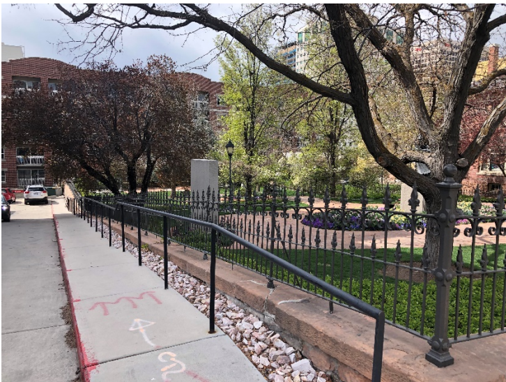
Existing fence along east property line
