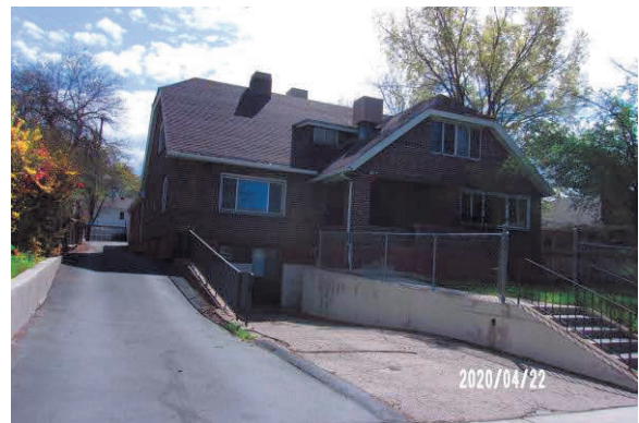
Southeasterly of West Building & Drive
