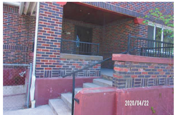
Main (Front) Entrance to West Building
