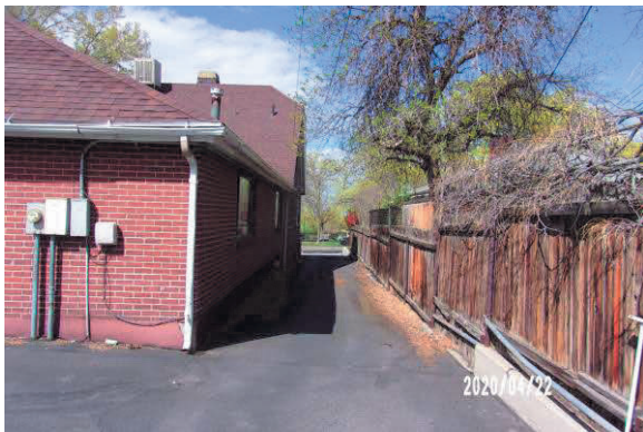
Westerly Along Drive (West Building)
