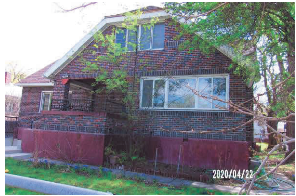
Northeasterly of West Building
