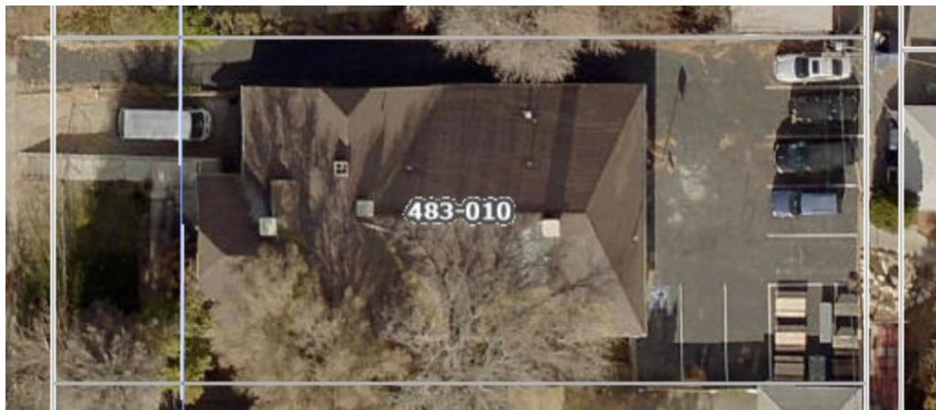
Figure 1 – Aerial photo of the property showing 8 parking stalls located on the rear of the lot.
