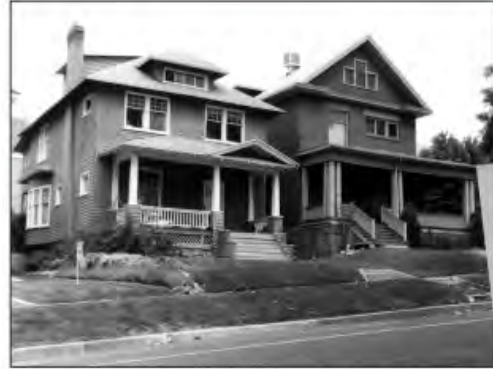
Because of its simplicity, the Foursquare lends itself to many styles. With thick square posts and exposed rafters it take on a Craftsman tone. With rounded porch columns and a pediment on the porch roof it becomes classical.
