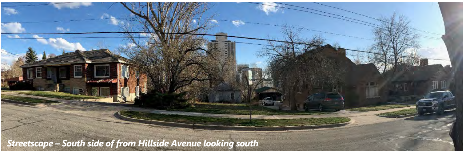
View of subject property from Hillside Avenue looking south
