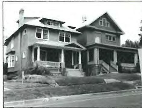
Because of its simplicity, the Foursquare lends itself to many styles. With thick square posts and exposed rafters it take on a Craftsman tone. With rounded porch columns and a pediment on the porch roof it becomes classical.
