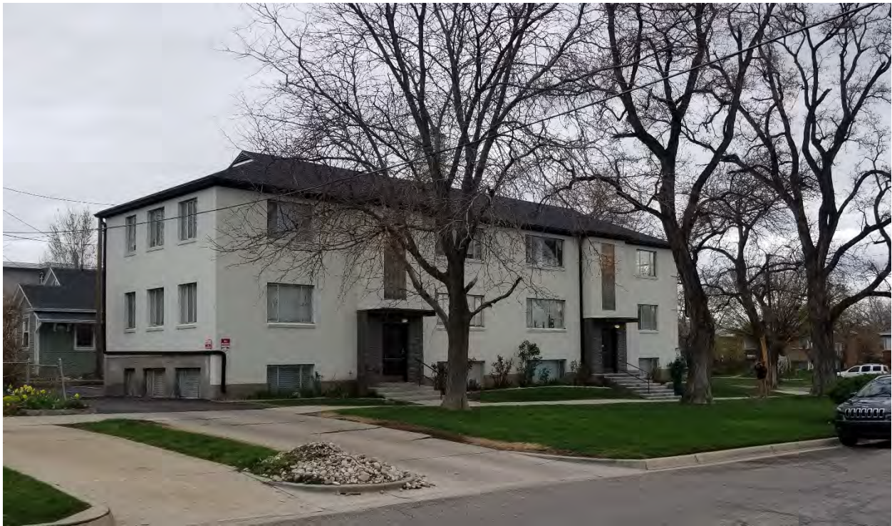
Image 9 – Current view of the building from 300 N shows the painted brick facades and painted stone entrances
