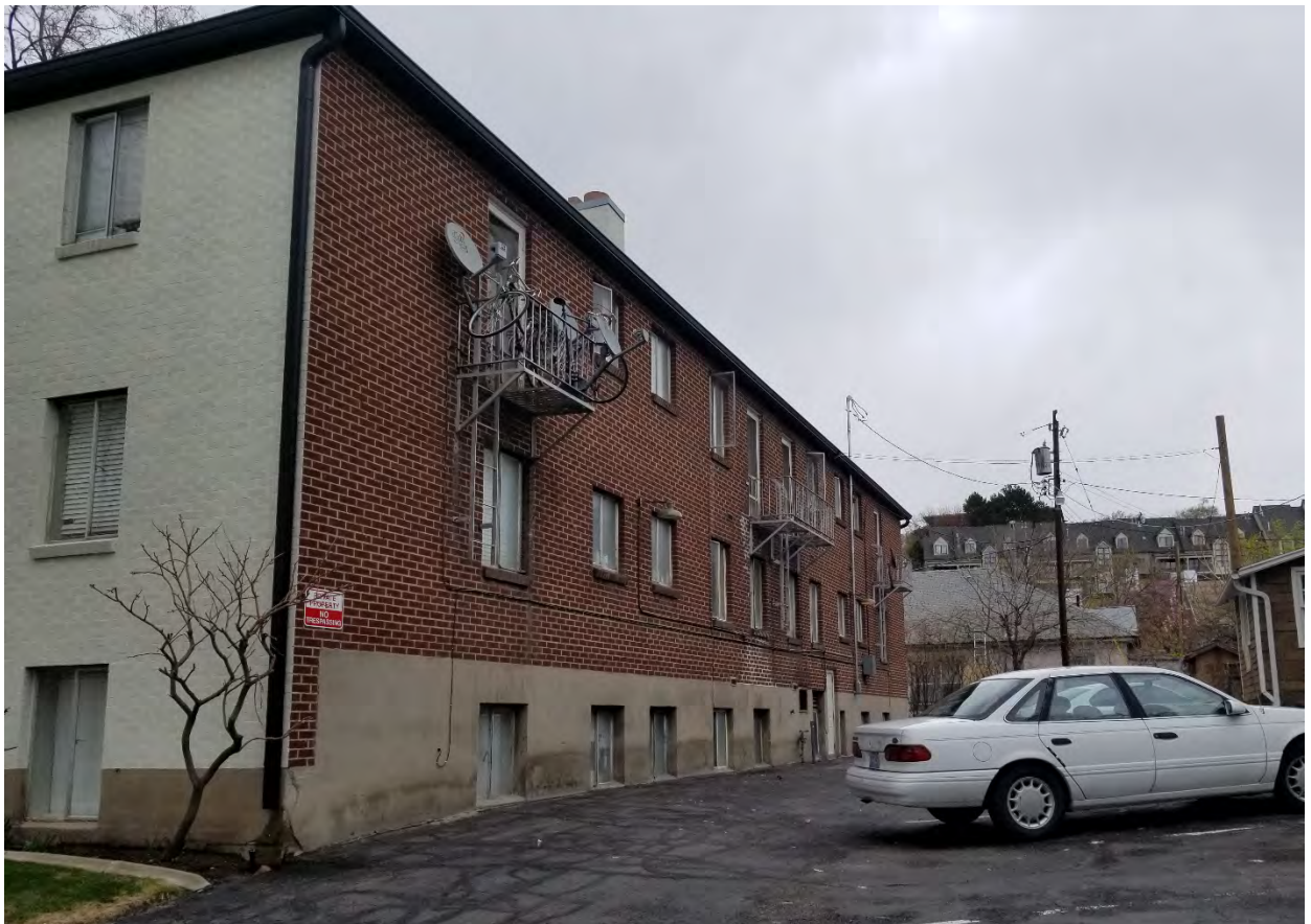
Image 12 – The rear (south) façade was left unpainted
