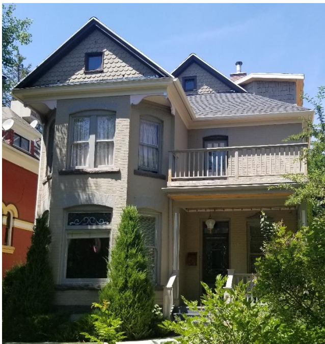
Figure 11 – New dormer is readily visible from the front façade of the home.
