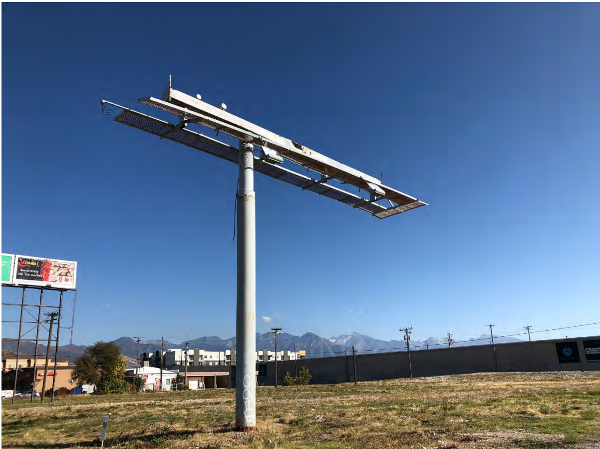
Existing billboard pole at approximately 643 S 400 West. View from 600 S looking south-east
