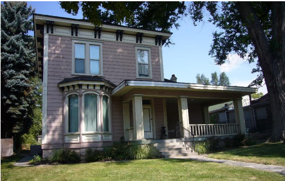
635 East 100 South (Landmark Building)
