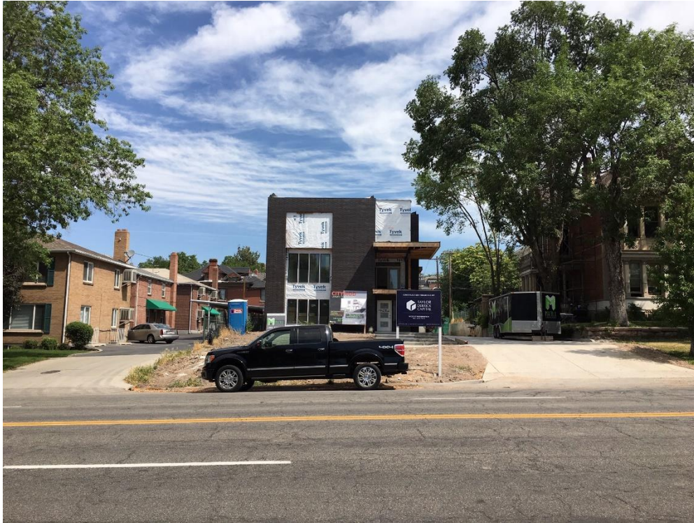
Subject Property Facing North
