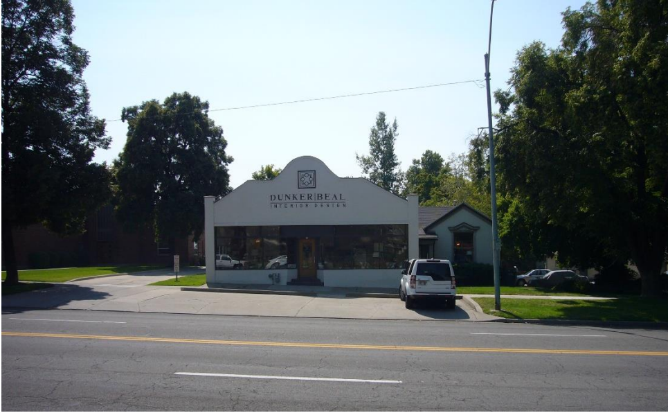
Commercial building across the street
