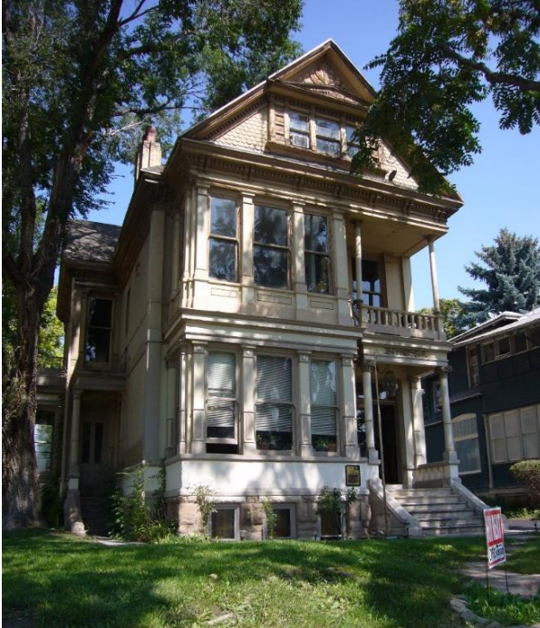
623 East 100 South (Landmark Building)
