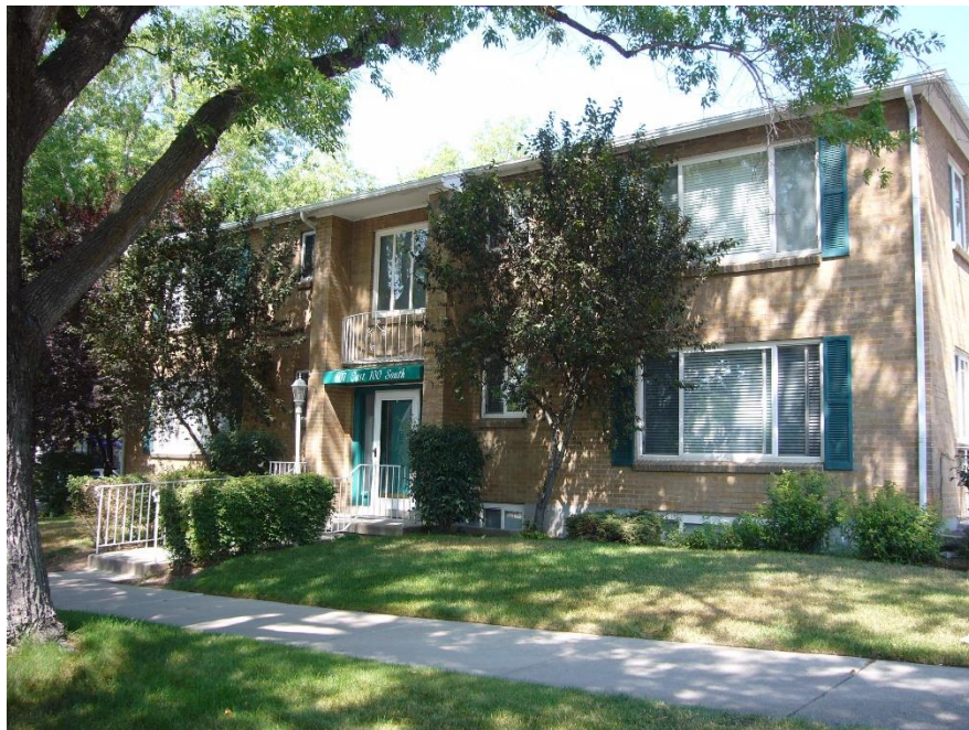
Property to the West
