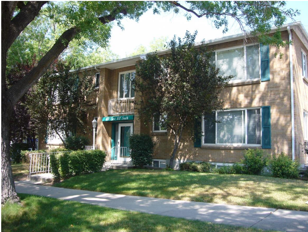
Apartment building to the west
