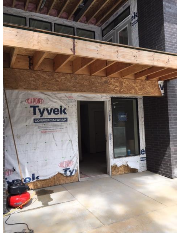
Entryway on East Façade
