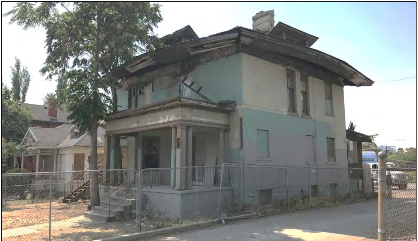
Street View of Subject Property (September 2017)
