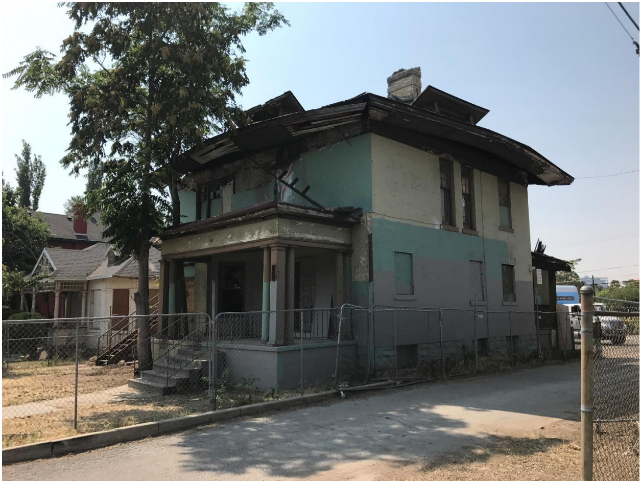
Photo of Building taken September 2016.
