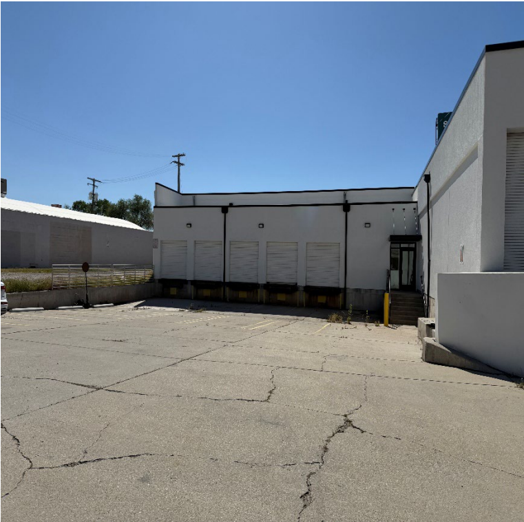
Subject property from the East (view from 500 W)
