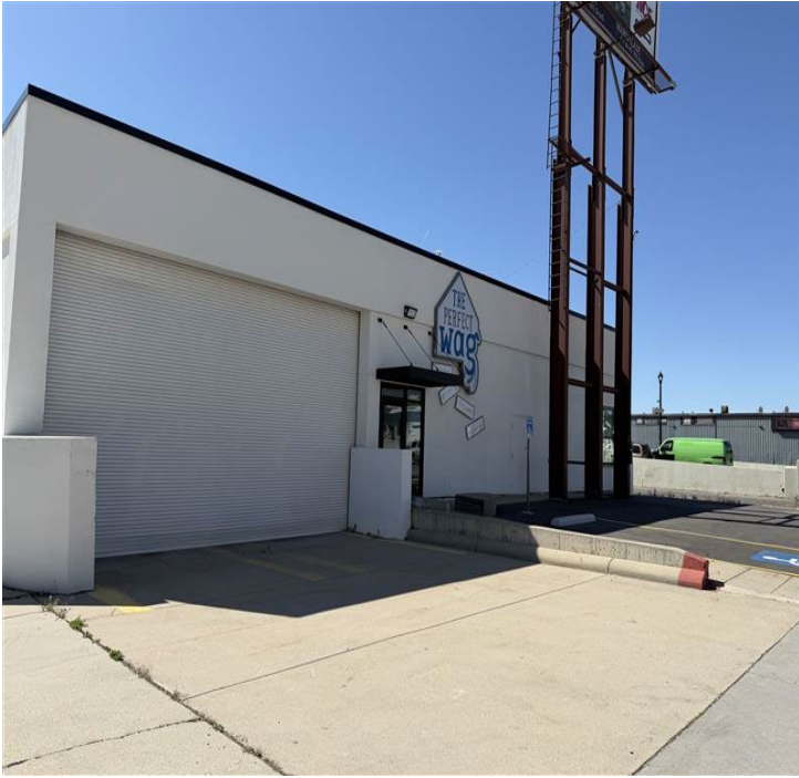
Subject property from the East (view from 500 W)
