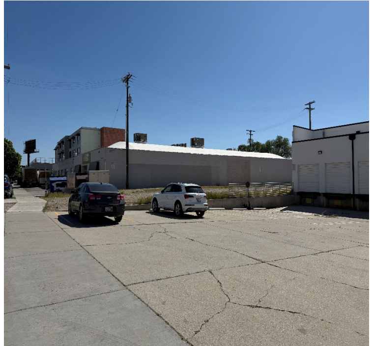
Subject property from the East (view from 500 W)
