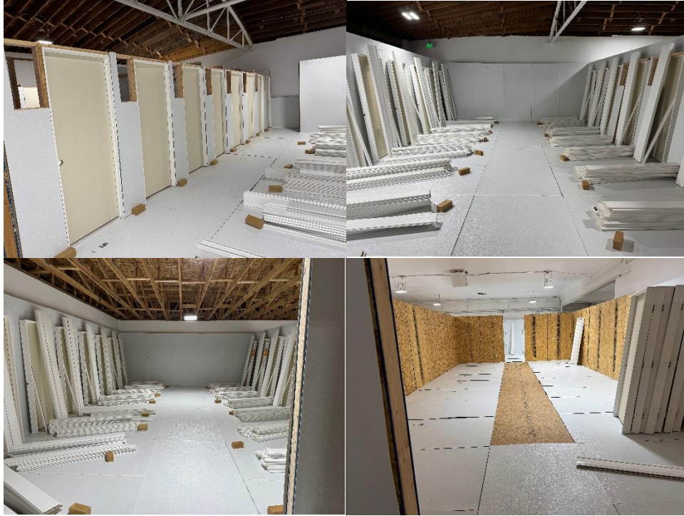
Pictures show in progress construction of individual rooms. 6 foot removable modular fencing is secured between each room and can be removed or added depending on the preference of the customer expanding space.
