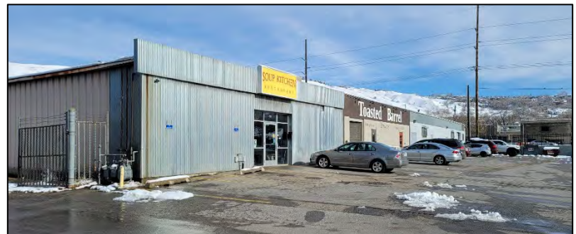
Front Façade of the Building viewed from the western side of the property
