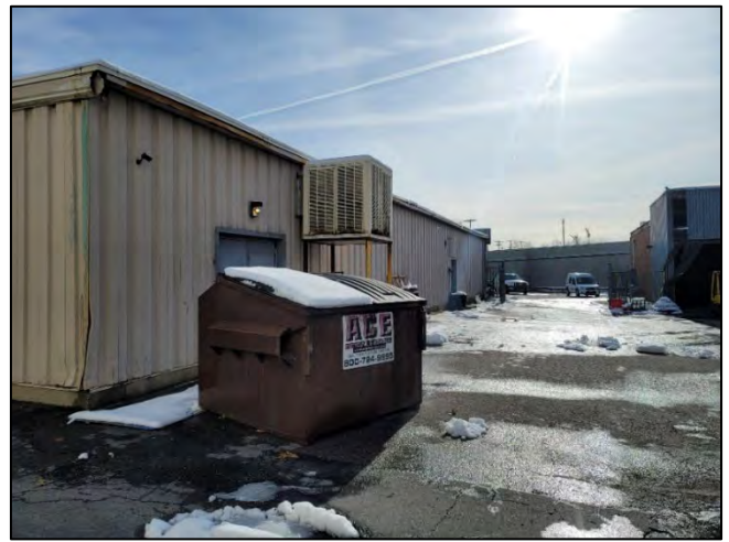
View of the western side of the building and dumpster
