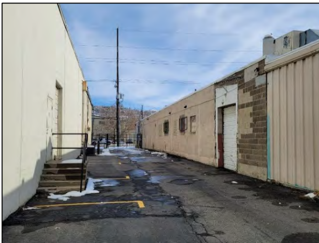
View of the rear façade of the building and neighboring building to the north
