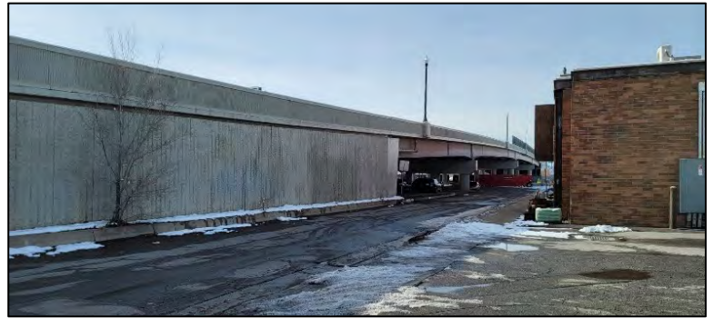
View to the west of the property of 600 North continue under the overpass
