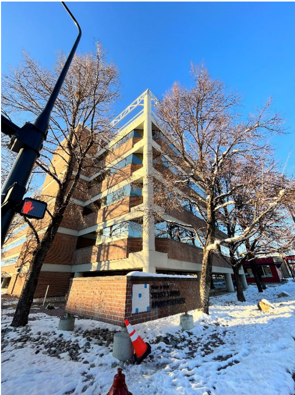
Xerox Building from corner of 500 S & 700 E
