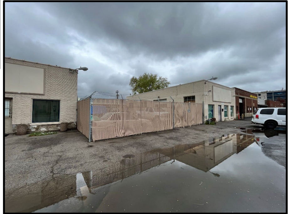
Subject site, facing southeast
