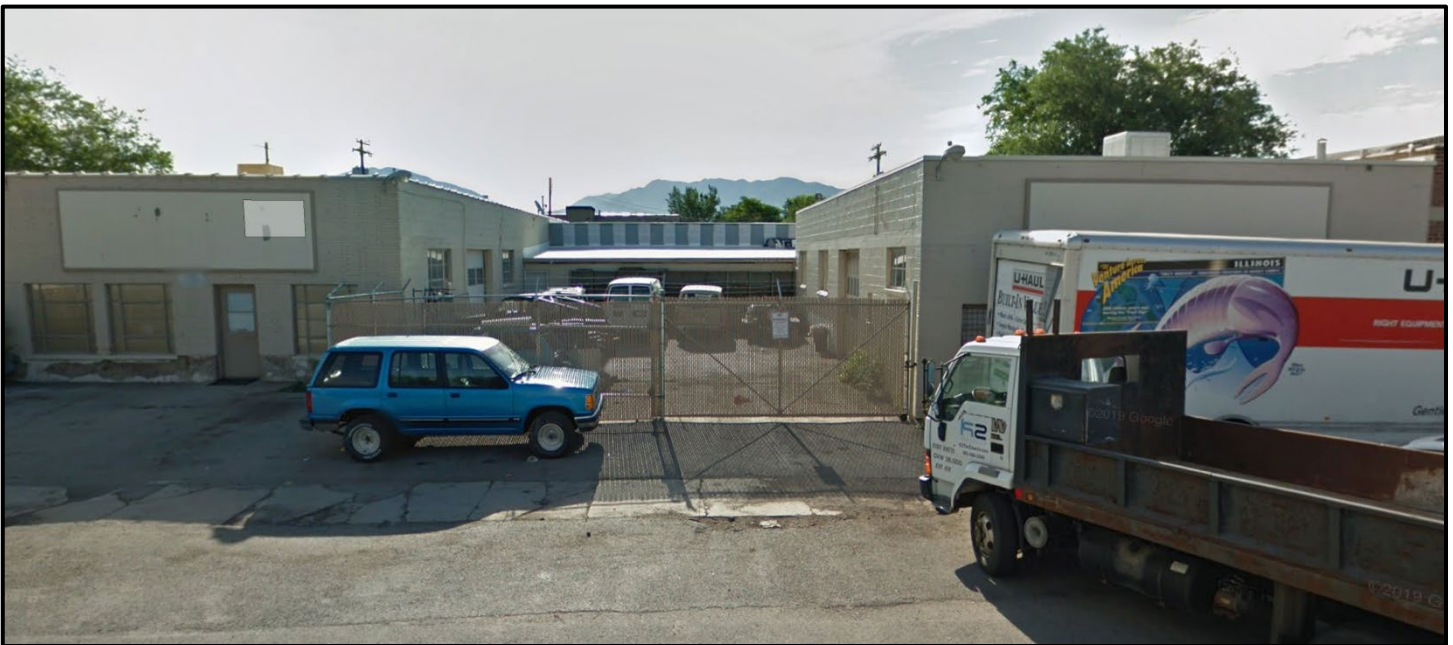
2011 Google Street View of the Subject Properties
