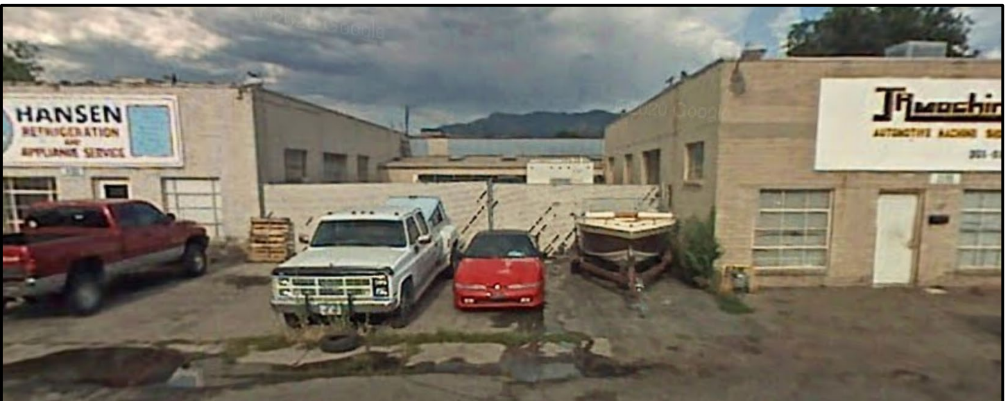
2007 Google Street View of the Subject Properties
